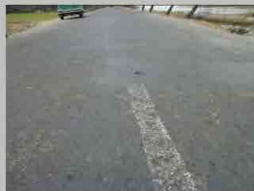
No. 4 Condition of road surface
