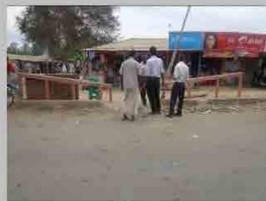
No. 4 Condition of road surface
