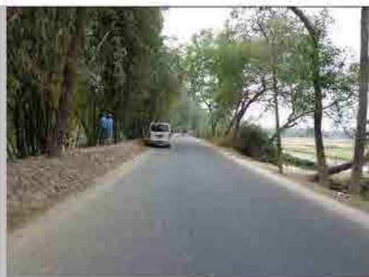
No. 1 Distance view to the forward
