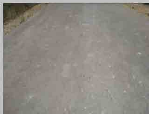
No. 4 Condition of road surface
