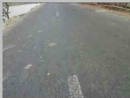
No. 4 Condition of road surface
