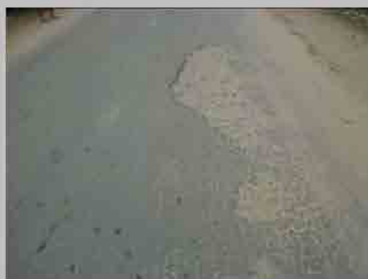
No. 4 Condition of road surface
