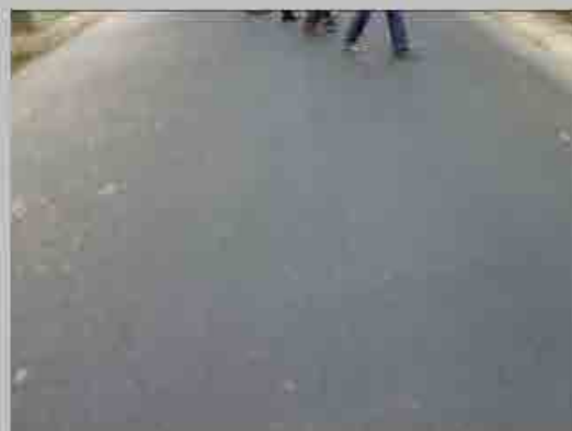
No. 4 Condition of road surface
