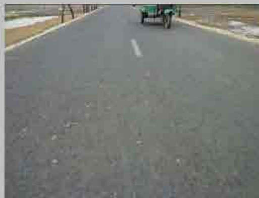
No. 4 Condition of road surface
