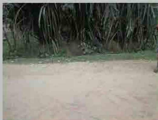
No. 4 Condition of road surface
