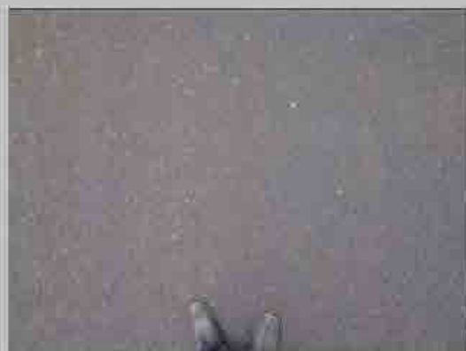
No. 4 Condition of road surface
