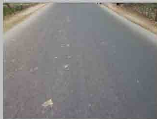
No. 4 Condition of road surface
