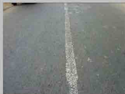
No. 4 Condition of road surface
