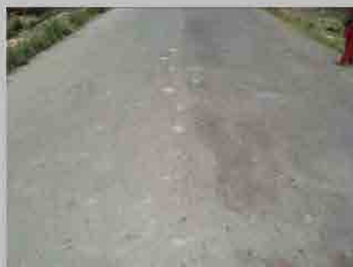
No. 4 Condition of road surface
