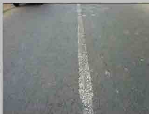
No. 4 Condition of road surface
