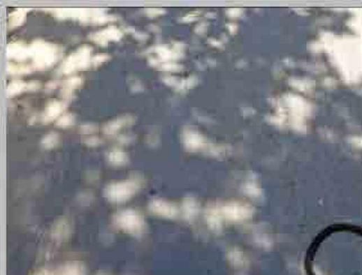
No. 4 Condition of road surface
