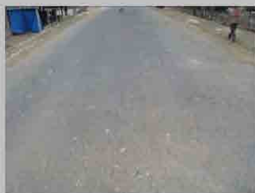
No. 4 Condition of road surface
