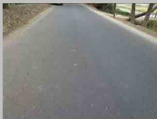
No. 4 Condition of road surface
