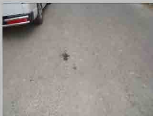
No. 4 Condition of road surface
