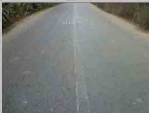
No. 4 Condition of road surface
