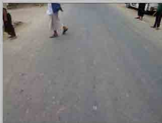
No. 4 Condition of road surface
