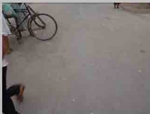
No. 4 Condition of road surface
