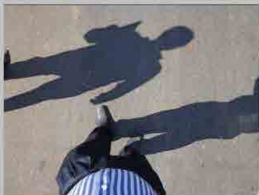
No. 4 Condition of road surface
