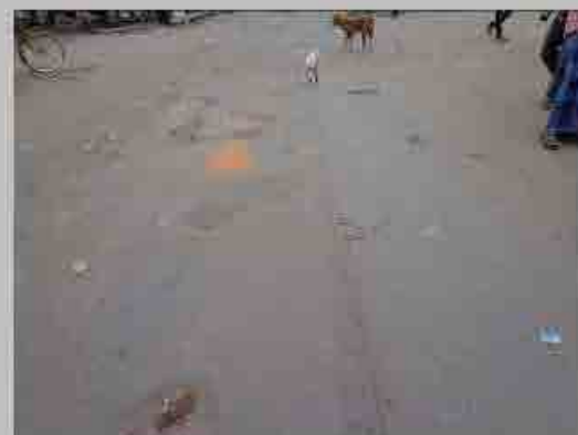
No. 4 Condition of road surface
