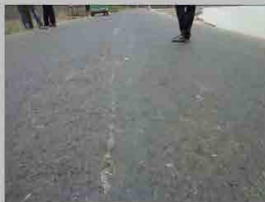
No. 4 Condition of road surface
