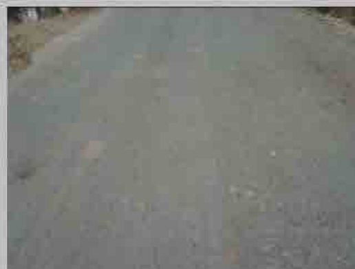
No. 4 Condition of road surface
