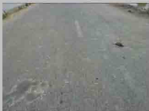
No. 4 Condition of road surface
