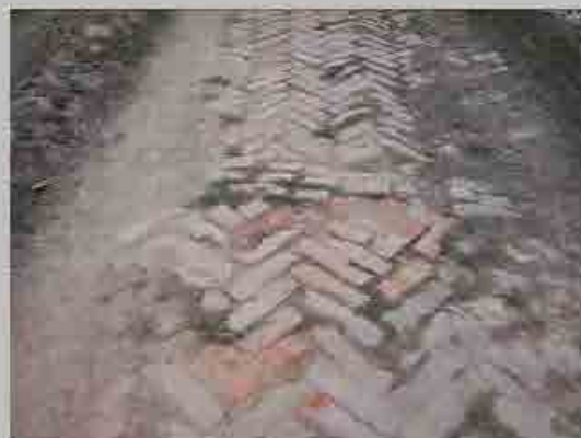
No. 4 Condition of road surface
