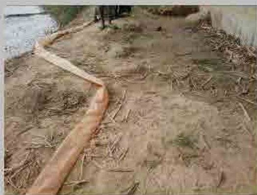
No. 4 Condition of road surface
