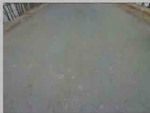
No. 4 Condition of road surface
