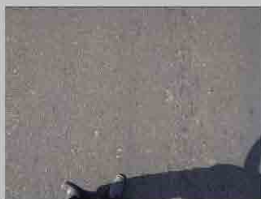
No. 4 Condition of road surface
