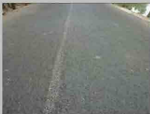
No. 4 Condition of road surface
