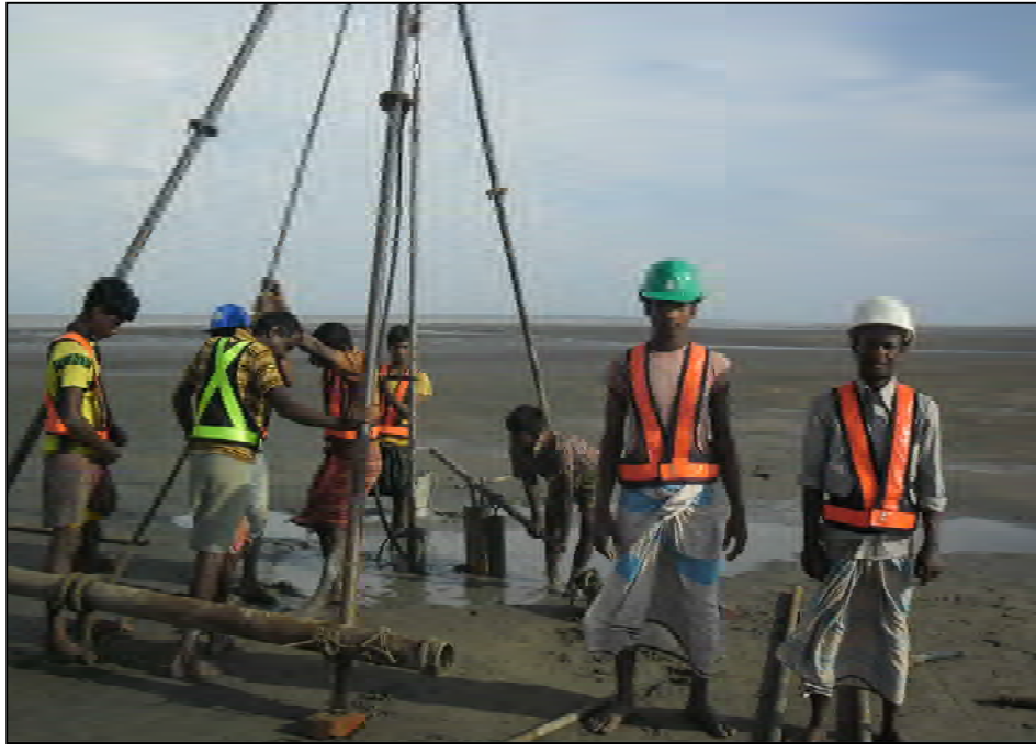
Figure -1 Soil boring at Matarbari site
