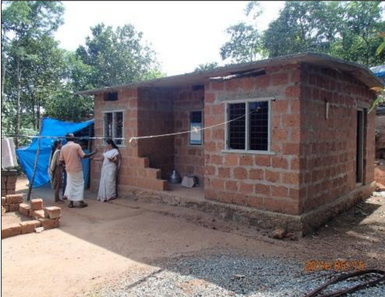
Community Infrastructure: House under construction in Ward 8, Thavinhal Grama Panchayat
