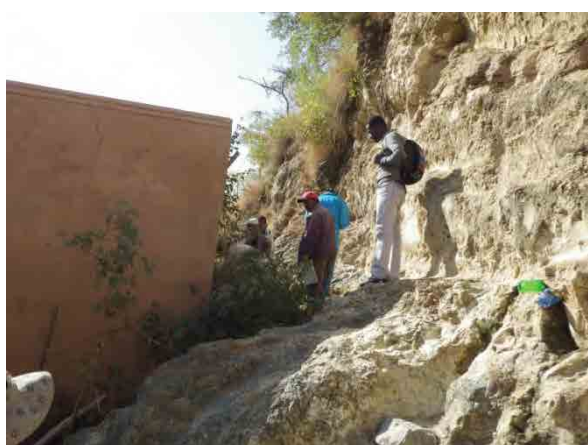
Steam bath house constructed closer to the cliff.
