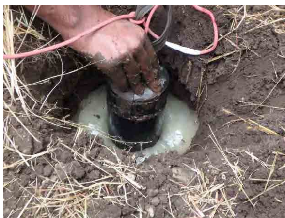
Setting of electrode below the ground
