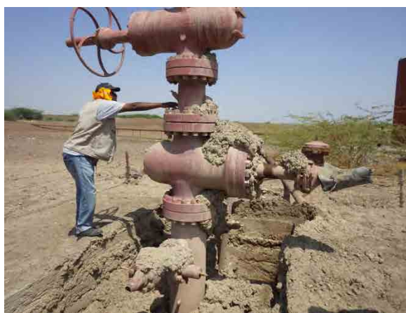
TD-4 Test well; mud is frown out beside the well.
