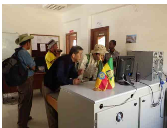
Operation room in Aluto-Langano Geothermal Power Plant
