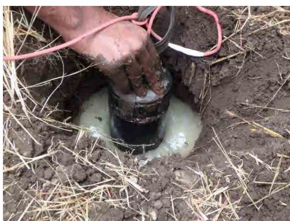
Setting of electrode below the ground
