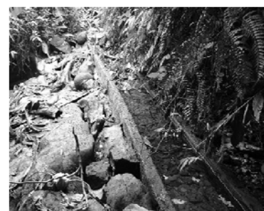
Canal Blocked with Landslide sediments
