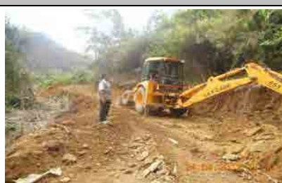
Construction of farm-link road
