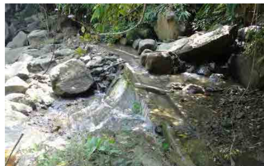
Photo 9.6.2 Typical Canal Sedimentation
