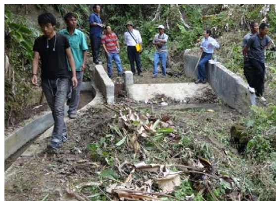
Typical Intake from Stream
