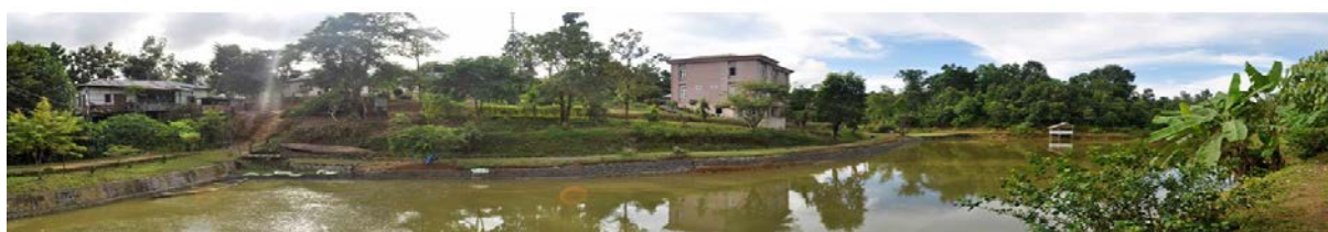
Northern view : Main Pond with Staff Quarters and Fish Farmers Training Center-cum-State Level Laboratory Building
