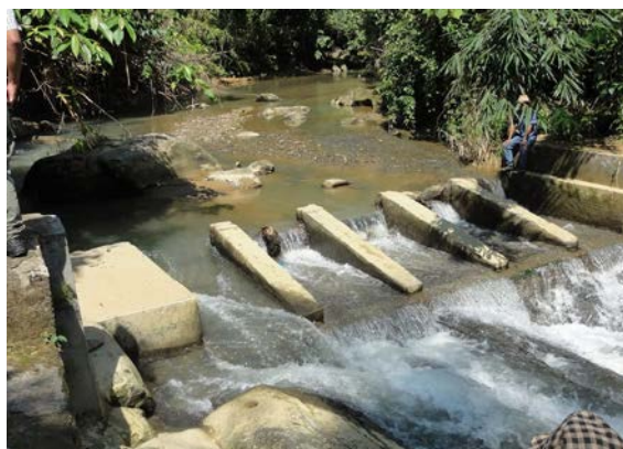
Typical Intake from Stream
