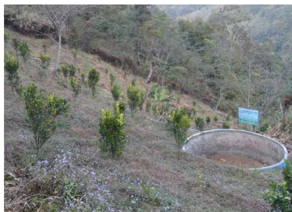
Water Storage Tank for Horticulture
