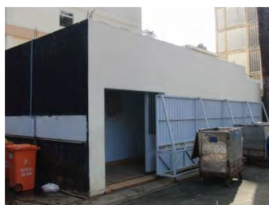
Figure 10-2 Infectious waste storage building
