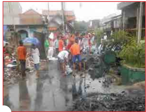
To put the land of sedimentation that has been dredged into the sacks by man power at PHB Klingkit, Rawa Buaya - Cengkareng
