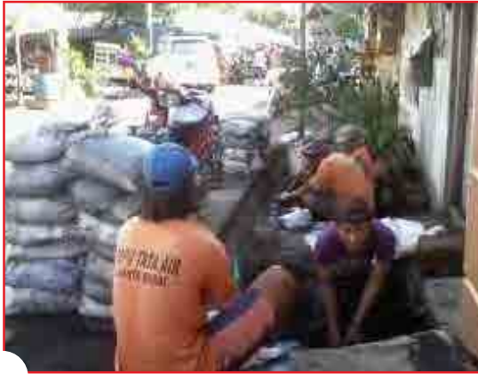
Excavation of sedimentation by man power at Jembatan Besi (Tambora)
