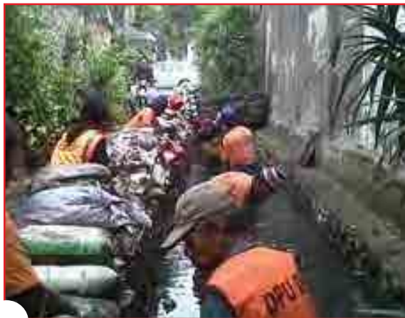
Excavation of sedimentation by man power at Saluran PHB Liberty (Tambora)
