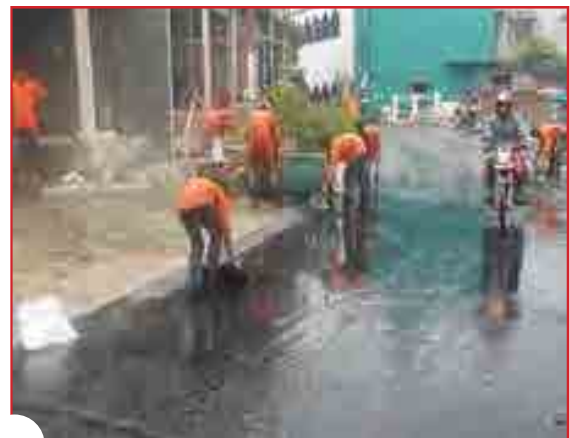
Road cleansing at PHB Klingkit, Rawa Buaya - Cengkareng
