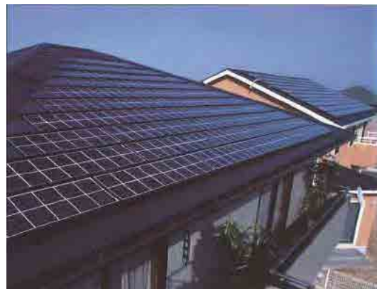
Figure 1-17 Examples of pitched roof installation
