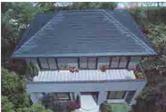
Figure 1-18 Examples of built-in module installation
