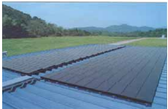
Figure 1-16 Example of deck roof installation
