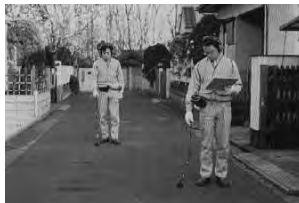
Detection Work by Water Leak Detector
