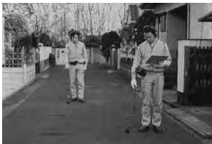
Detection Work by Leak Detector
