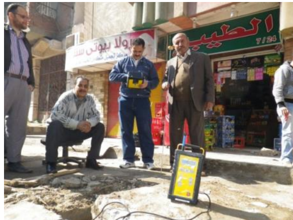
Figure 4.2-4 Leak Noise Correlator Survey on GHAPWASCO
