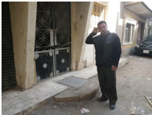
Figure 4.2-13 House Connection Survey using Acoustic Rod on MCWW
