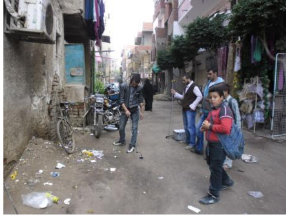
Figure 4.2-15 Ground Surface Survey using Water Leak Detector on MCWW
