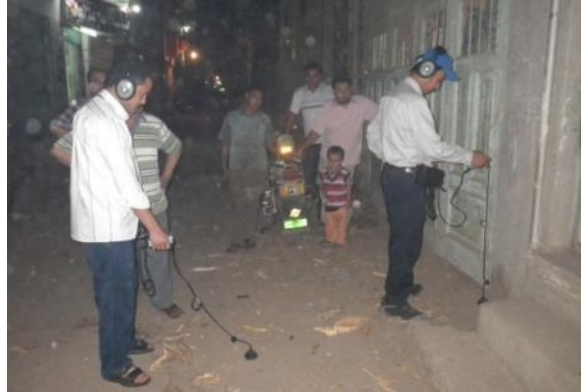
Figure 4.2-5 Ground Surface Survey using Water Leak Detector on GHAPWASCO
