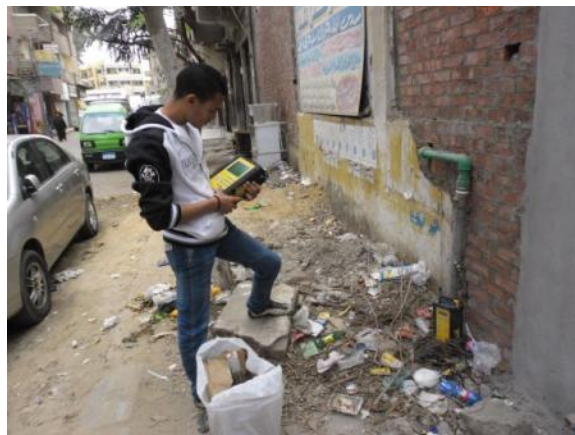
Figure 4.2-14 Leak Noise Correlator Survey on MCWW
