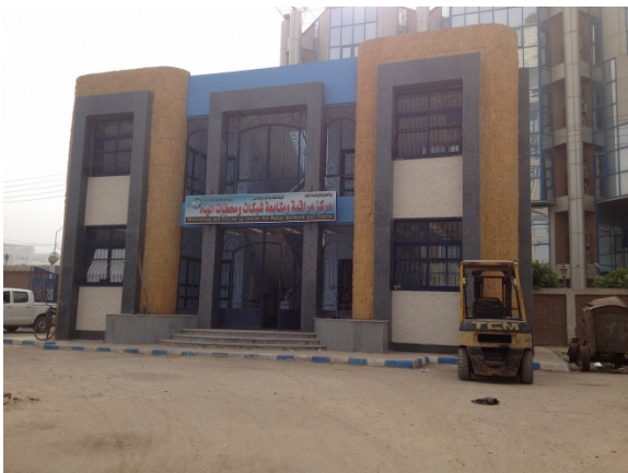
Central monitoring room, constructed by SHAPWASCO, March 2014
