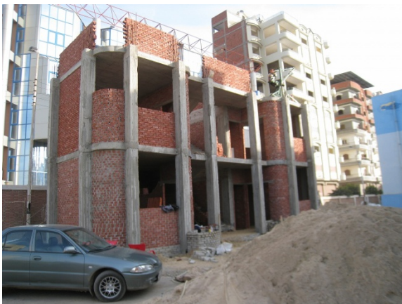
WDM monitoring room under construction, February 2013
