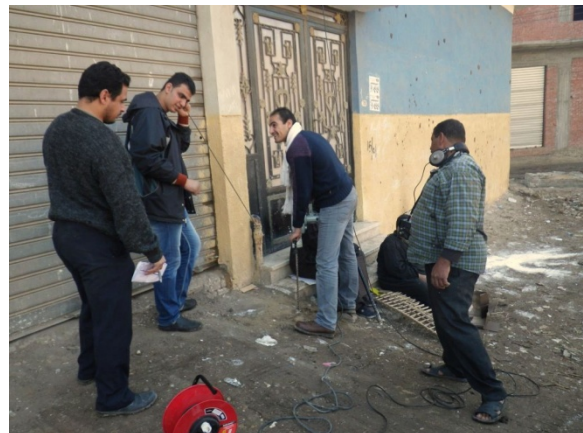
Confirmation work of leakage in Quesna Markaz, February 2013
