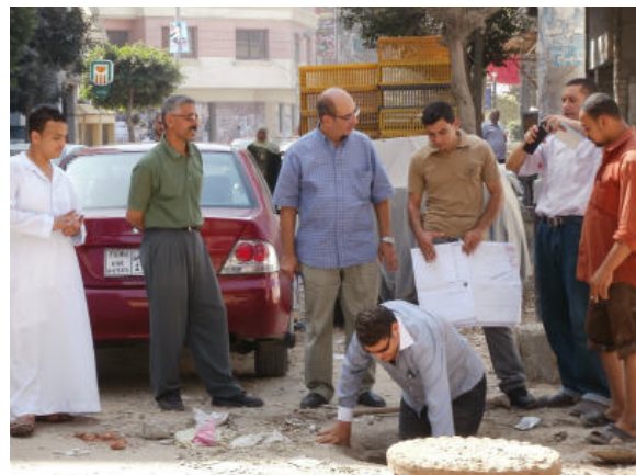
Site confirmation of valve condition, October 2011
