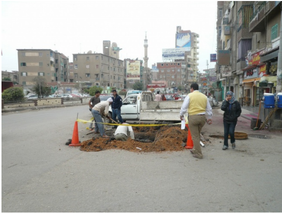
Construction of chamber for water flow meter, December 2012
