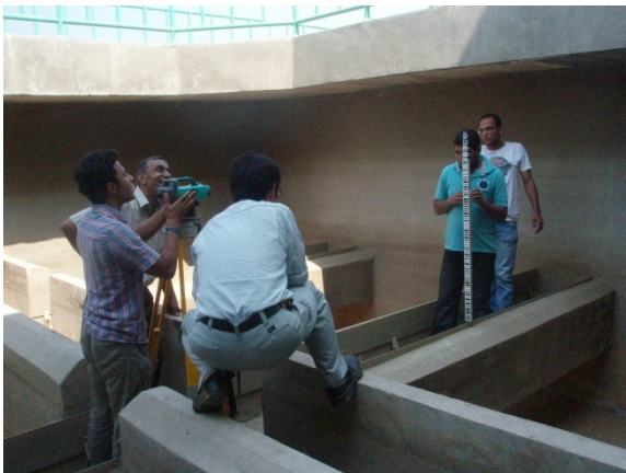
Level adjustment of collecting trough, Tanta El Teraa El Melahia SWTP, October 2012
