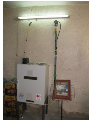
Installation of pressure gauge for pressure monitoring, May 2013
