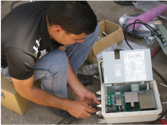
Installation and setting of water flow meter, May 2013
