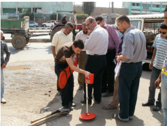
Confirmation of location for pipeline, October 2011
