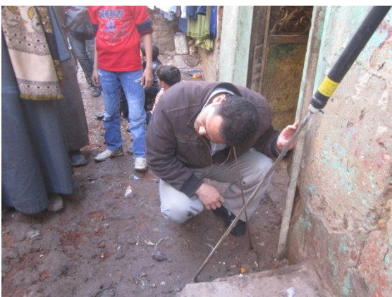
Confirmation work of leakage in Zefta Markaz, January 2013
