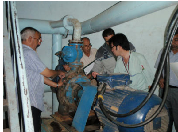
Confirmation works for current condition of water supply facilities, October 2011
