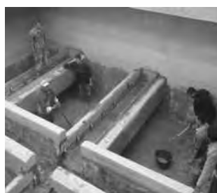
ADJUSTING FILTERS SAND LEVEL
