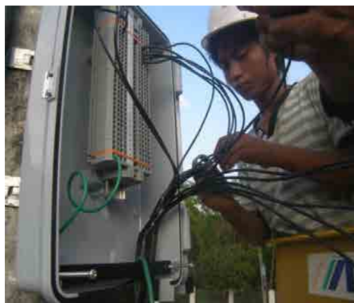
端子箱配線中
