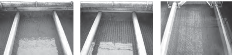
Figure 3.1-8 Condition of Tube Settler
