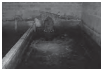
Source: JICA Survey Team Original Clear Water Well constructed in 1970s Inflow from Filter
