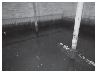
Original Clear Water Well Ground water penetrates into the decrepit well from outside when water level in the well is lower.
