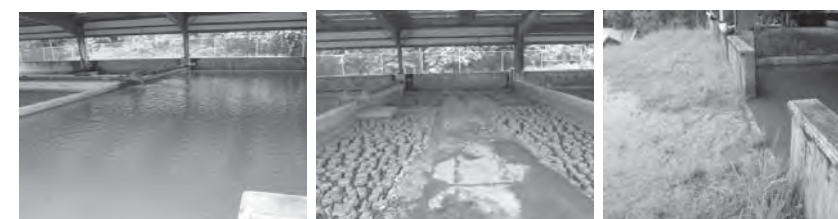
Figure 3.1-12 Sludge Drying Bed
