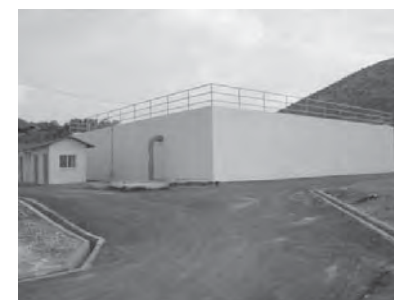
Figure 3.3-7 Rectangular Reinforced Concrete Tank (sample)
