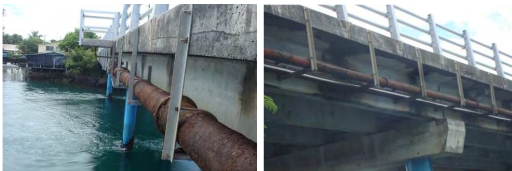
[Left] West Side of Minatobashi Bridge and Existing Sewer, [Right] East Side of Minatobashi Bridge and Existing Water Distribution Pipes (DN4in: 100mm x 2)
