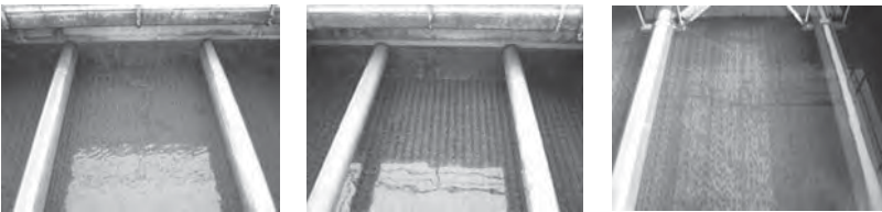
Figure 3.1-8 Condition of Tube Settler
