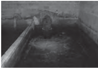
Source: JICA Survey Team Original Clear Water Well constructed in 1970s Inflow from Filter
