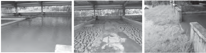
Figure 3.1-12 Sludge Drying Bed
