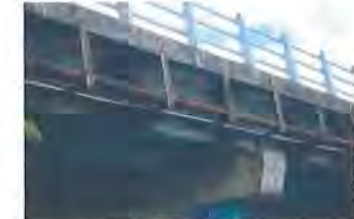
Minato-bashi (East side: Long Island side) : Existing water pipeline (dia. 4" x 2 lines)
