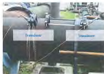
Installed on pipe from raw water pump at KAWTP
