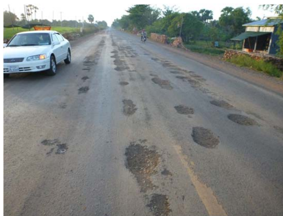
Figure 6 Damaged Pavement
