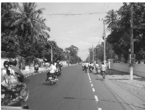
Photo 4.1-1 Edge Line and Paved Shoulder
