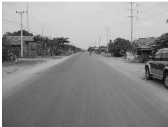
Photo 4.1-2 Roadside Higher than Road Surface without Drainage
