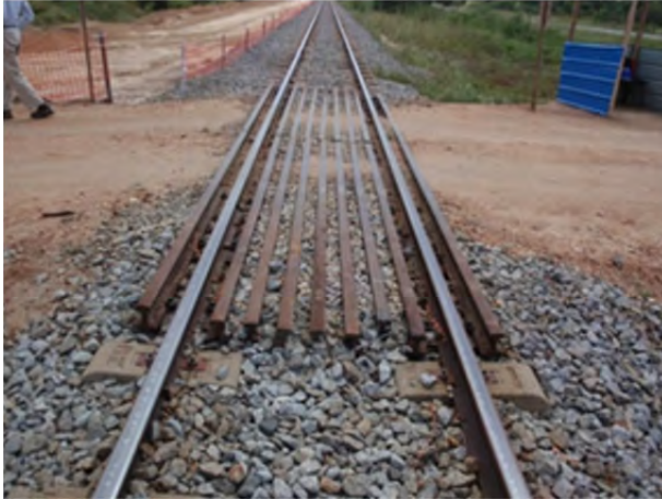
Figure 2-20 Actual railway crossing
