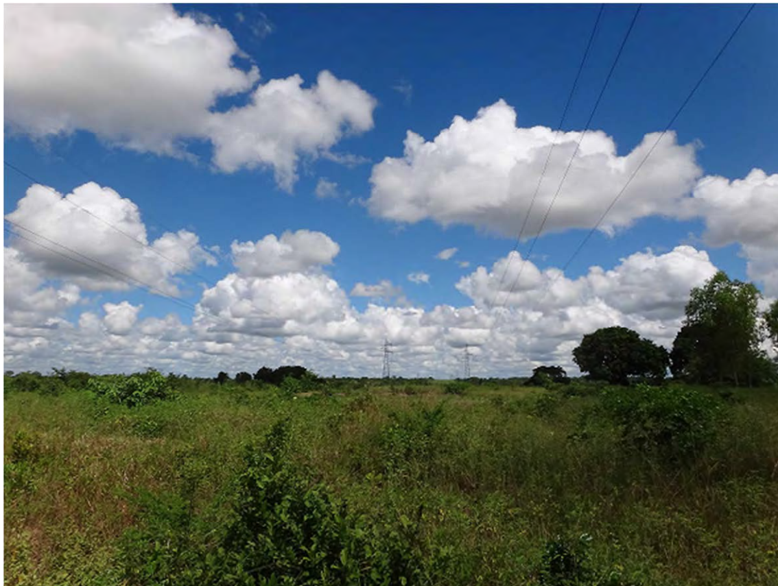
Figure 2-2 Overall view of the Namialo substation construction site
