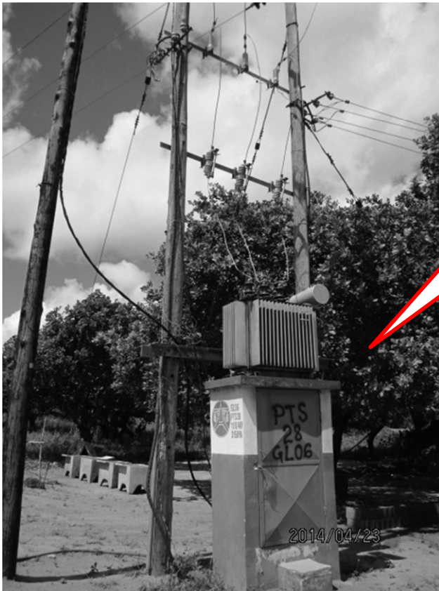
Figure 2-13 Installation image of a 33kV distribution transformer
