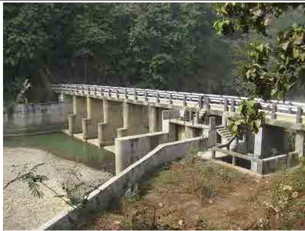
Chathe Minor Irrigation Project (Dimapur)
