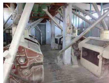
Source: JICA Survey Team Flour Mill in Industrial Estate
