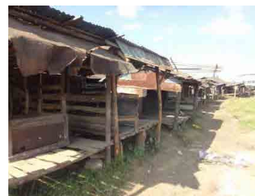
Source: JICA Survey Team Rural Market Sheds (Jaintia Hills)
