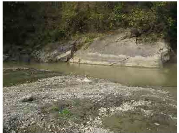
Dzuza Medium Irrigation Project (Dimapur)
