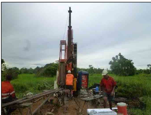
Figure 4.1: GDI drilling rig used during the investigations.
