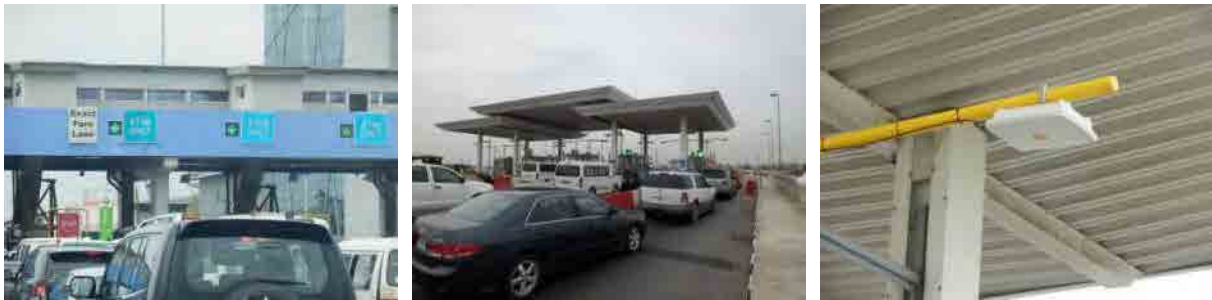
ETC Gate (Lekki-Epe Expressway) ETC Gate (Lekki-Epe Expressway) Antenna for ETC (Lekki-Ikoyi Bridge)
