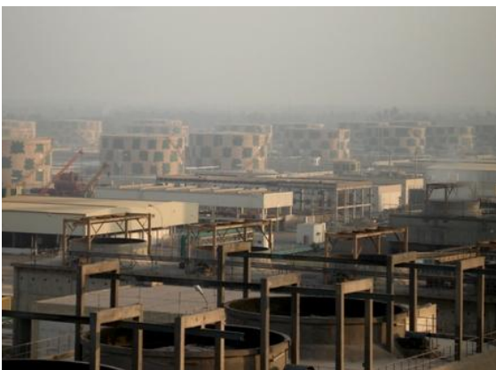
Photo 5-5 Cooling towers and oil tanks
