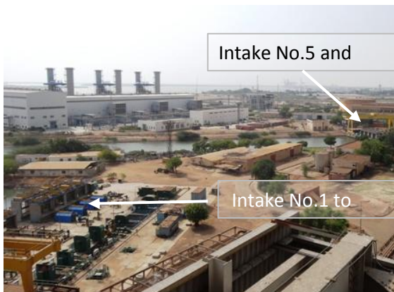
Photo 1-5 Intake of cooling water
