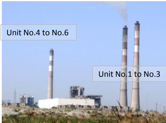
Photo 2-1 Full view of the power station
