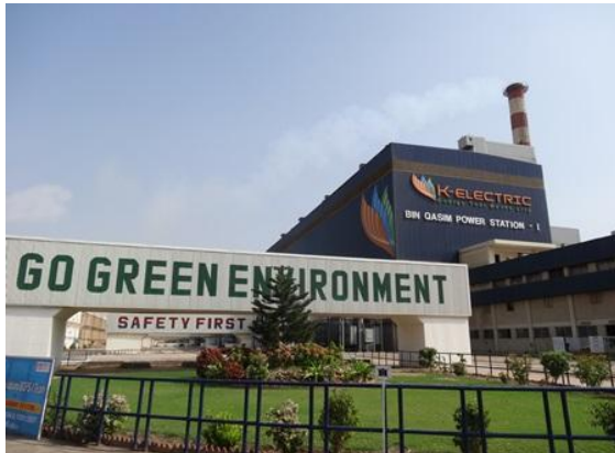
Photo 1-1 Main Building from entrance gate
