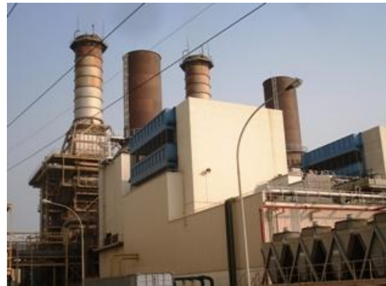
Photo 5-2 Steam turbine building (front)
