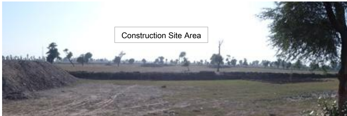
Photo 8-1 Sahiwal Power Plant Project Site1
