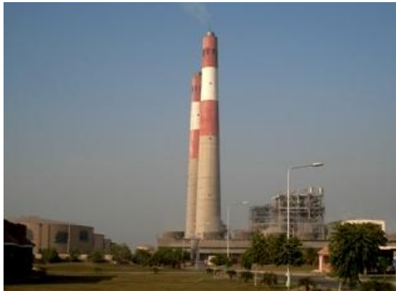
Photo 6-1 Full view of the power station
