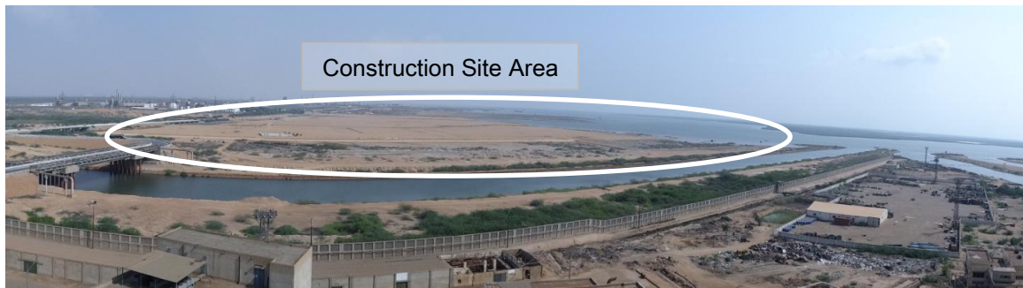
Photo 8-3 Port Qasim Power Plant Site
