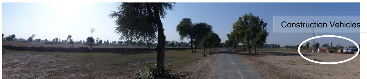
Photo 8-2 Sahiwal Power Plant Project Site2
