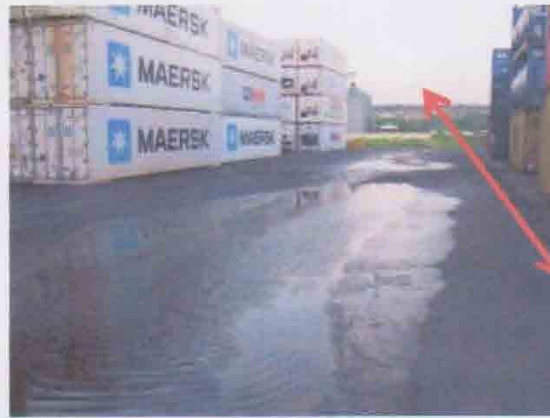
Photo-① Settlement behind the rear wall (2013 April)
