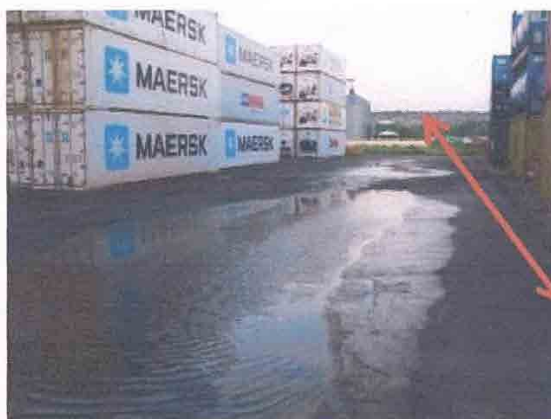
Photo-① Settlement behind the rear wall (2013 April)
