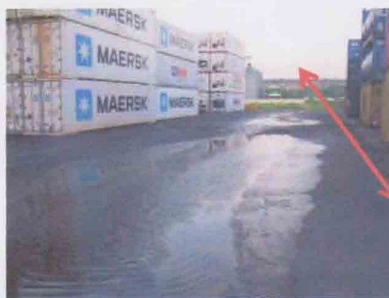
Photo-① Settlement behind the rear wall (2013 April)
