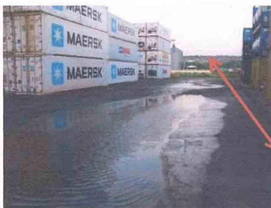
Photo-① Settlement behind the rear wall (2013 April)
