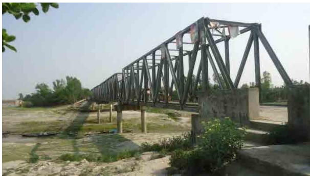
Figure 1.4 Kazirhat Bridge site
