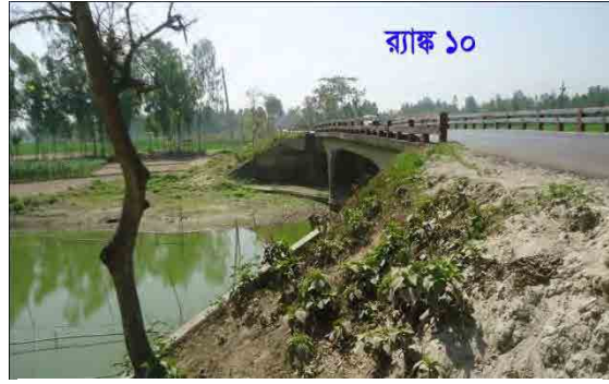
Bupibath bridge-Rank-10, Gaibandha
