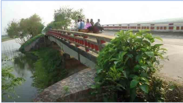
Figure 1.2 Mohasthan Bridge site
