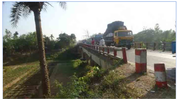
Figure 1.3 Chanda Bridge site
