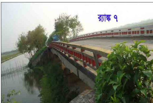
Chanda Bridge-2, Rank-7, Sirajganj
