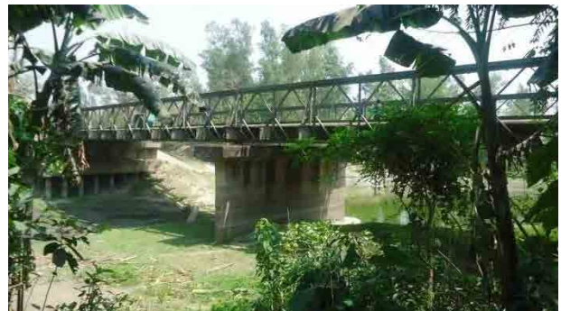
Figure 1.5 Naiori Bridge site
