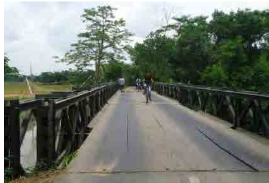
Paprail Baily bridge- Rank-77, Shariatpur
