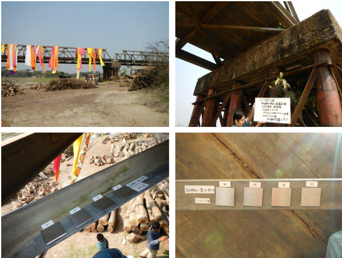
Figure 8.4.4 Installation of Exposure Test Specimens at Existing Bridges
