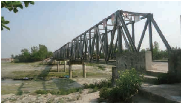
Figure 1.4 Kazirhat Bridge site
