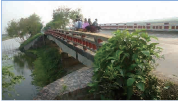
Figure 1.2 Mohasthan Bridge site
