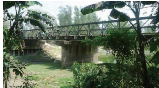
Figure 1.5 Naiori Bridge site
