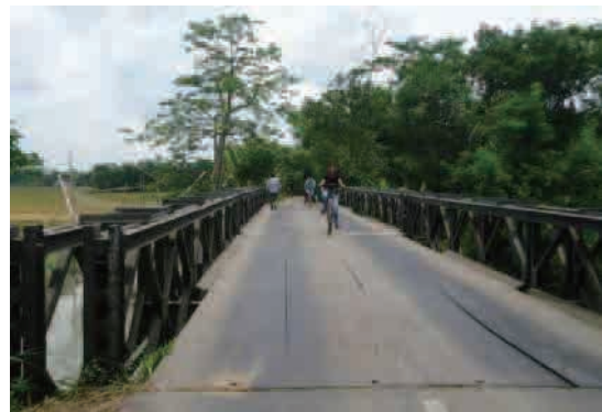
Paprail Baily bridge- Rank-77, Shariatpur
