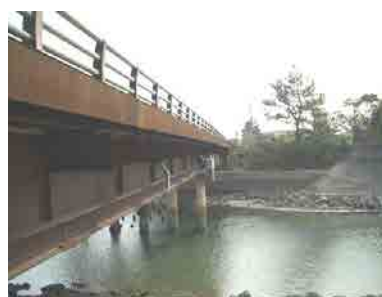
Name: Chita second bridge , Location: Handa city, Aichi Pref.
