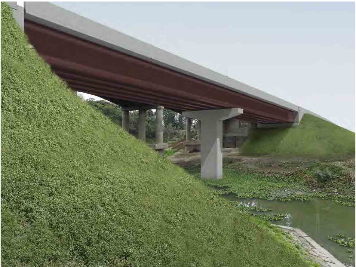
View of Steel-I Girder Bridge
