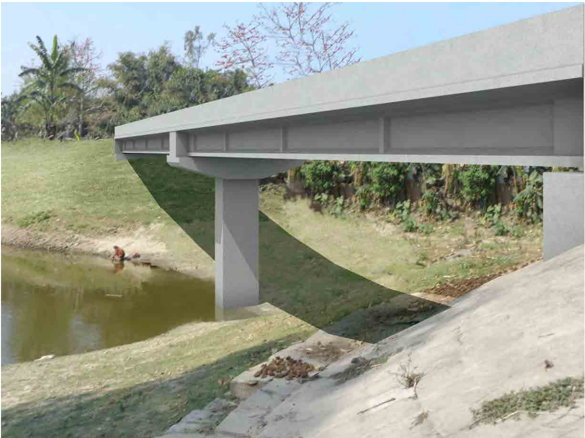
View of PC-I Girder Bridge
