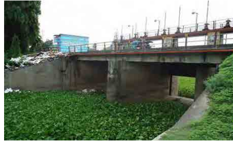
Bridge Integrated with Sluice Gate
