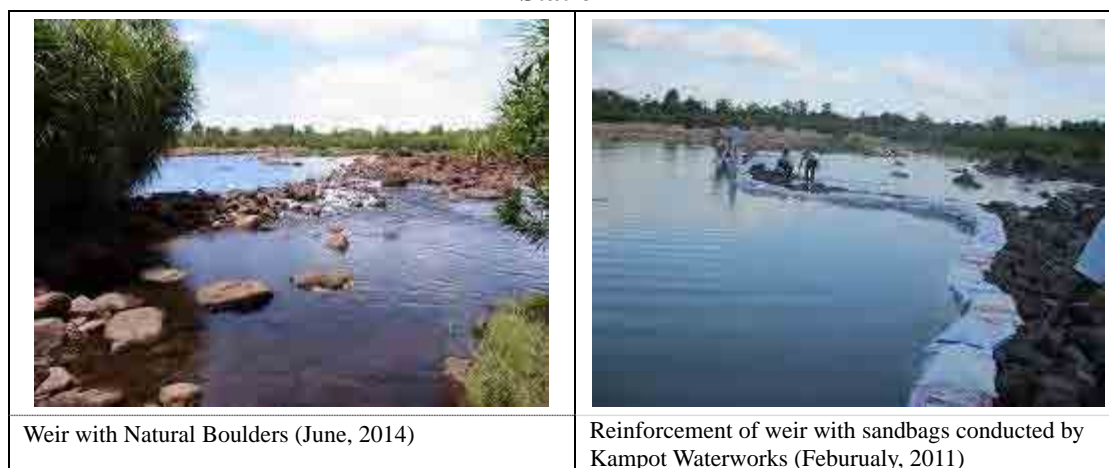
Photo 2.2.2.2-2 Weir with Natural Boulders Located Downstream of the Existing Intake Station
