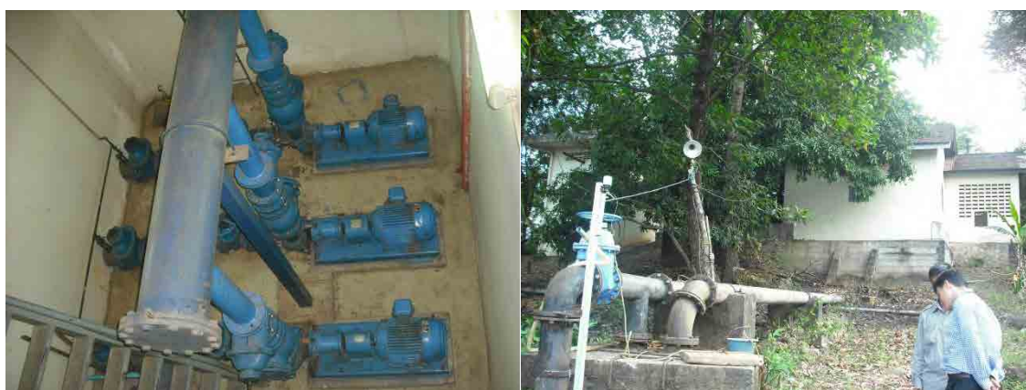
Photo 1.4.5-3 Condition of Existing Facilities
