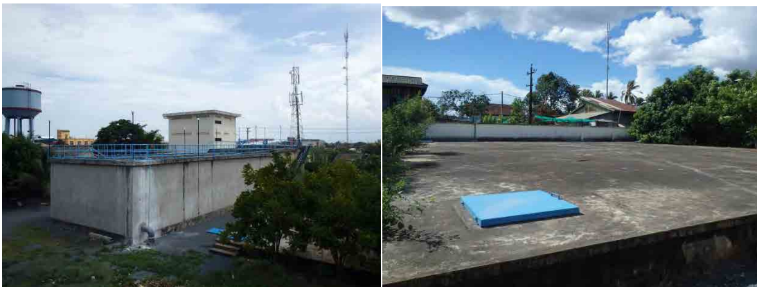
(left) Rapid Sand Filter (Right) Treated Water Reservoir
