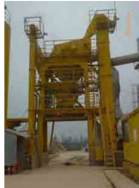
General view of the asphalt plant
