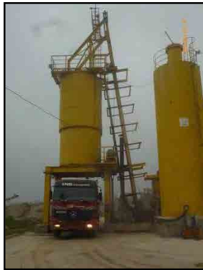
Loading onto a dump truck under the surge bin
