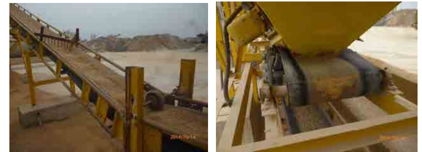
Pushing roller at the bending corner and large block removing device
