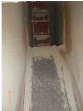
Buckets of Filler elevator and upper shoot
