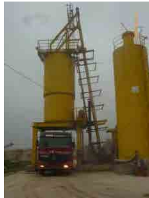
General view of surge bin
