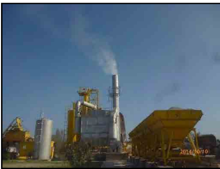
Dust from the chimney due to damaged cloths of bag filter
