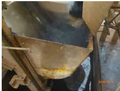
Asphalt mixture is just put in the bucket of Skip.
