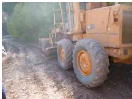
Photo3-2 Maintenance work of a regional road (Debar)
