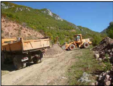
Wheel loader at site
