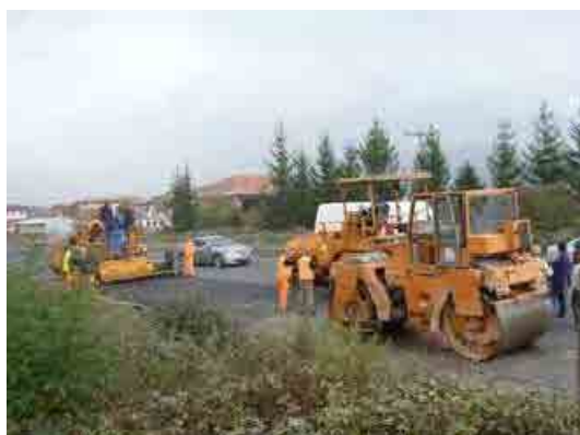
Photo3-1 Maintenance work of a magistral road (Bitola)
