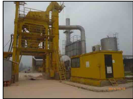
Asphalt plant and control room
