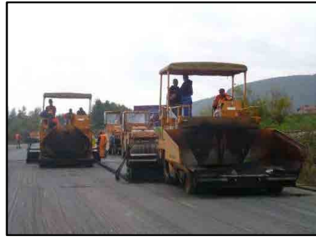
Paving work by procured equipment
