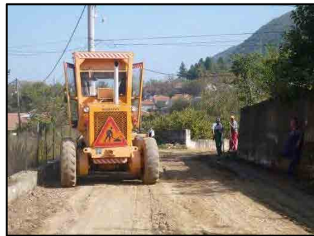
Motor grader at site
