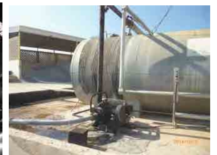
Locally replaced gear pump at the ground
