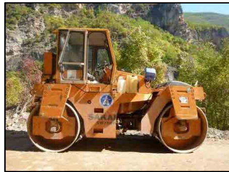
10ton Vibration roller at site
