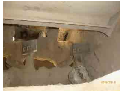
Inside Mixer (No wear at rotating wings and so on)
