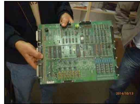
Damaged control panel board by lightning
