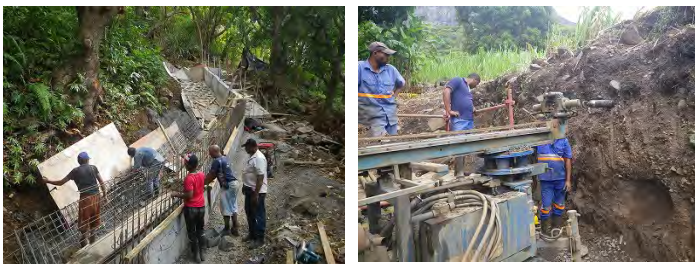
Construction work (left: new channel, right: horizontal drainage)
