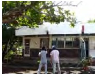
Checking of the damaged houses at site
