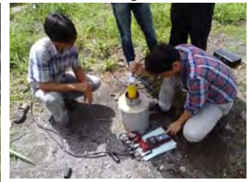
Monitoring of slip surface movement (by borehole inclinometer)
