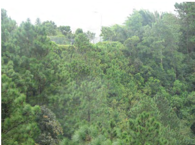
Full view of the slope failure
