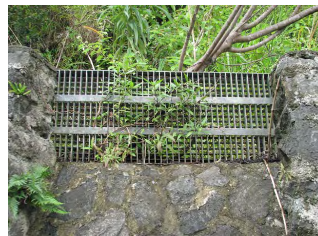
Outlet of surface water on the slope
