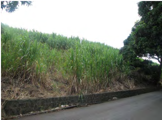
Full view of the slope
