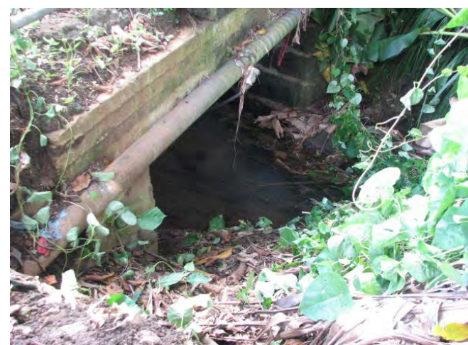
Inlet of box culvert
