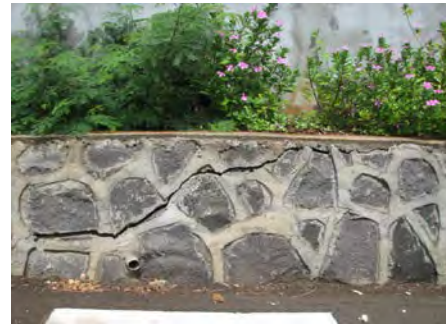
Cracks on stone wall
