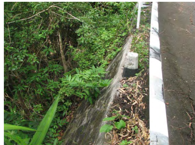
Retaining wall of the road along A-A' line
