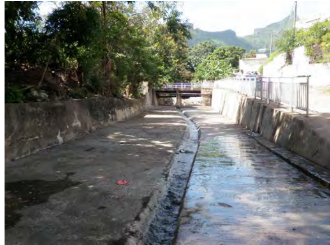
Full view of the channel (Upstream)
