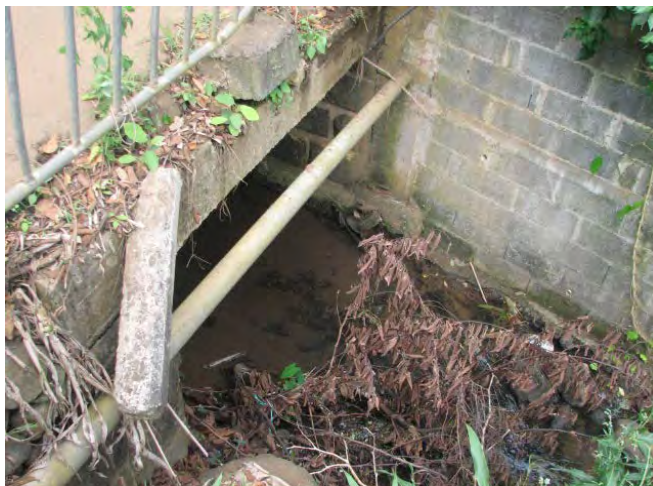
Outlet of box culvert
