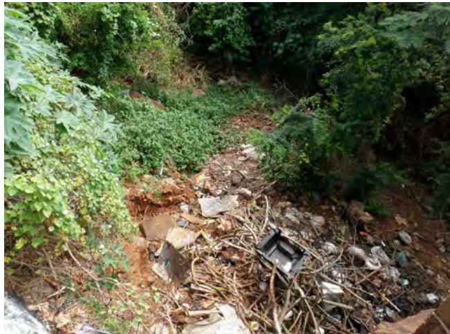
Bank erosion around bridge abutment
