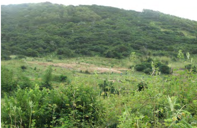
Upperpart of the landslide
