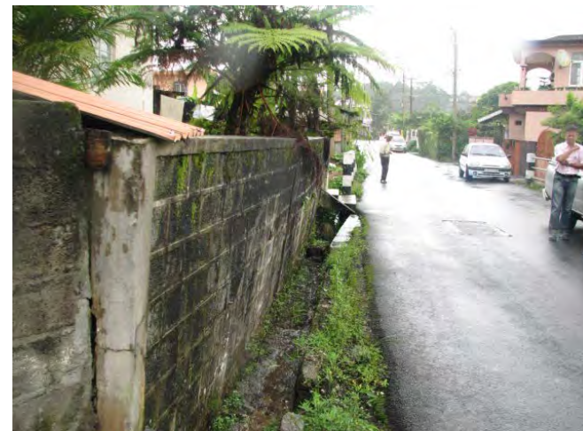
The inclined concrete block wall
