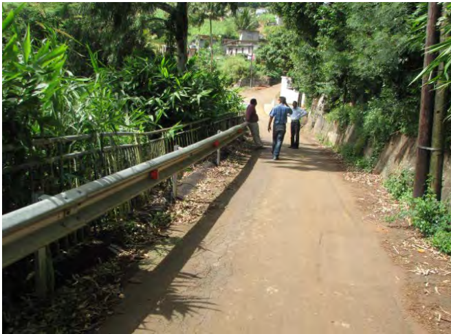
Full view of the road
