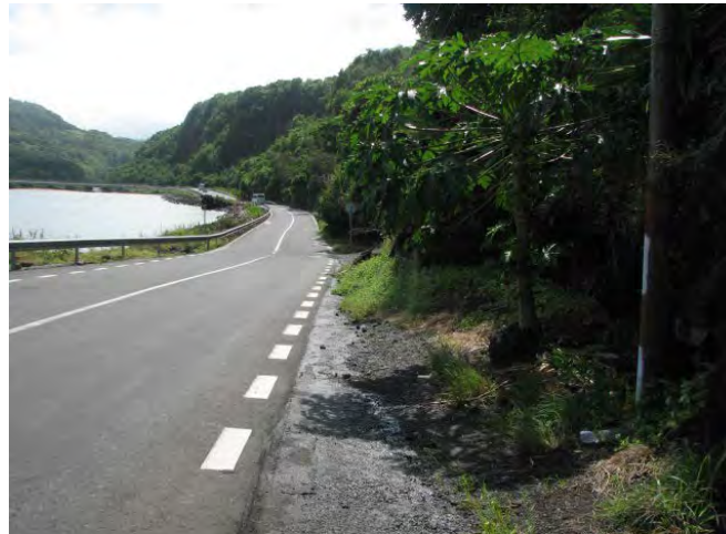
Clearance of the slope 2
