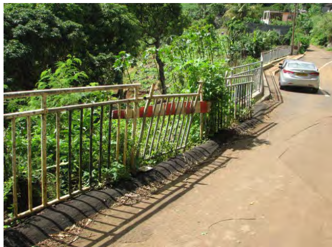
Repaired road of another site
