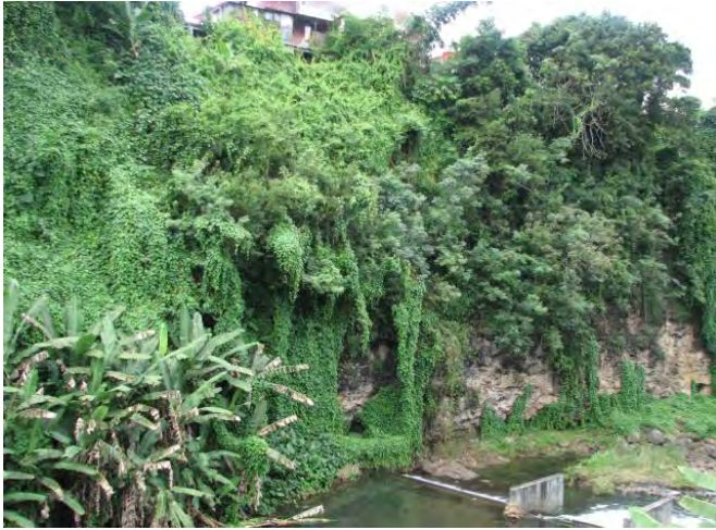
Full view of the slope from opposite side
