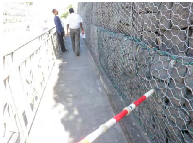
Gabion reinforced with rust prevention wire net
