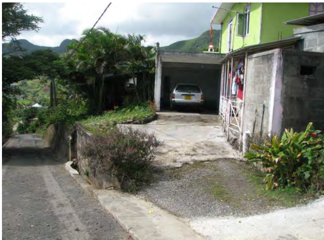
Full view of concrete block wall
