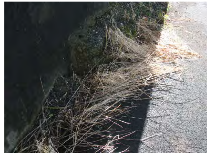
Spring water point (no water at the inspection)
