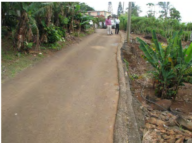
Retaining wall that comes off
