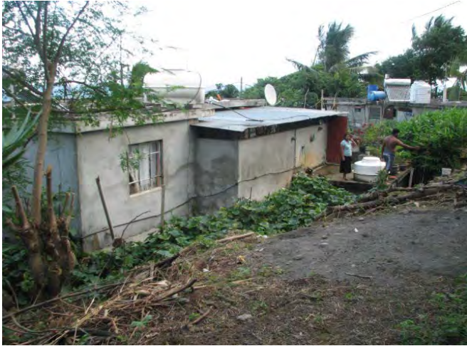
Full view of the slope and house
