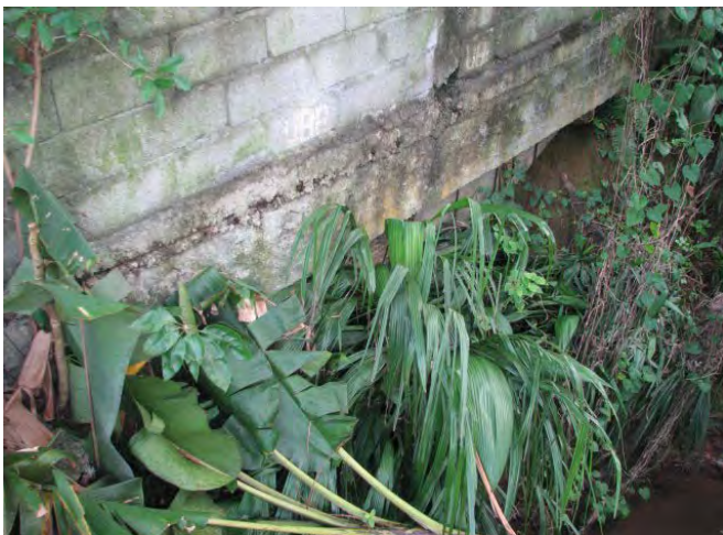
Outlet of box culvert
