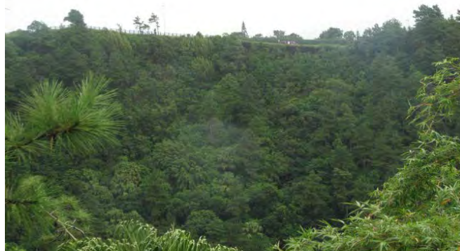
Full view of the slope failure Vegetation is getting recovery
