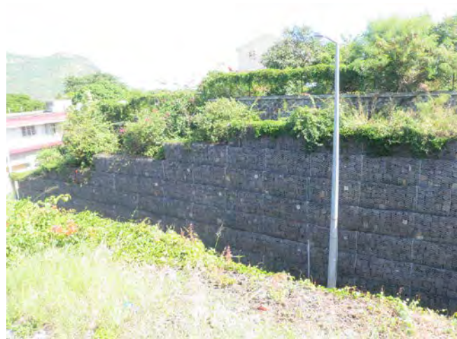
Full view of Gabion wall (West side)
