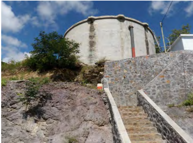
Full view of the slope from road
