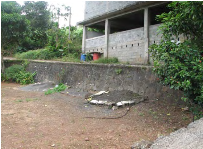
Full view of the retaining wall
