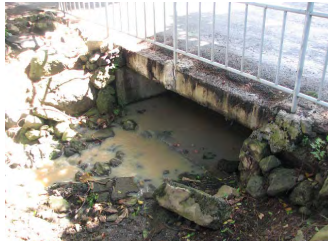
Outlet of the box culvert
