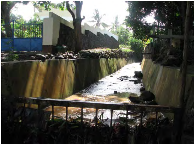
Full view of the channel work
