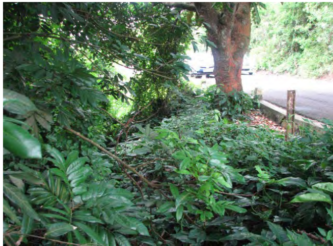
Slope under the shoulder
