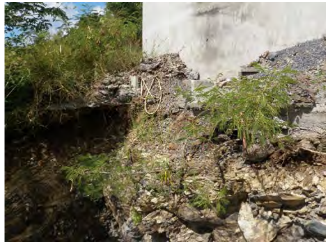
Outcrop of tank foundation
