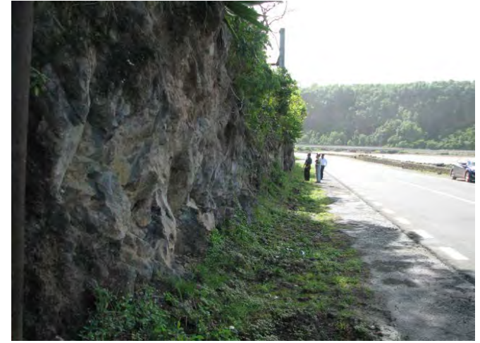
Clearance of the slope 1
