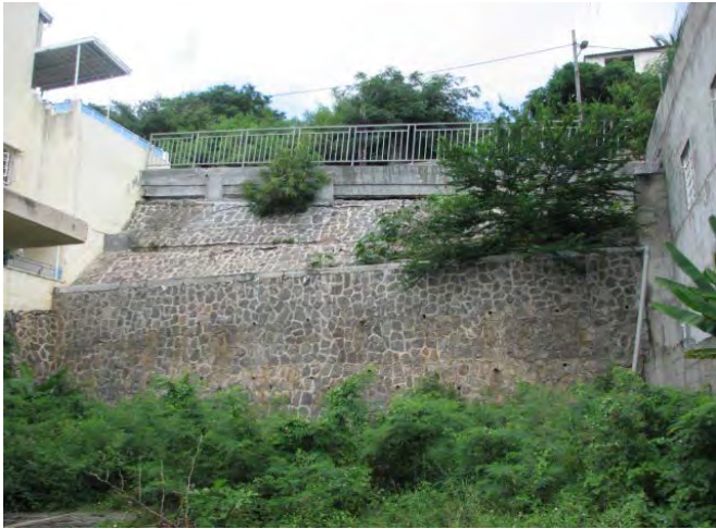
Full view (retaining wall)
