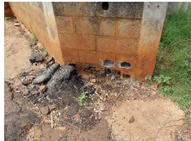
Grinding hole for drain.
