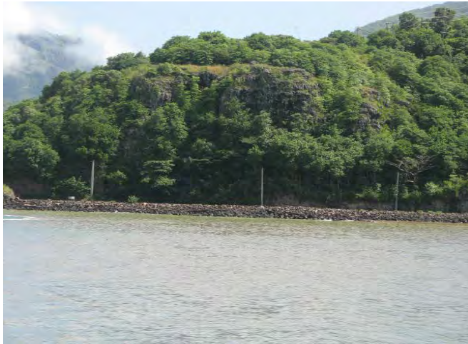
Full view of the slope 1
