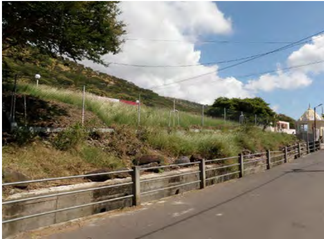
Slope in the retaining wall upper part
