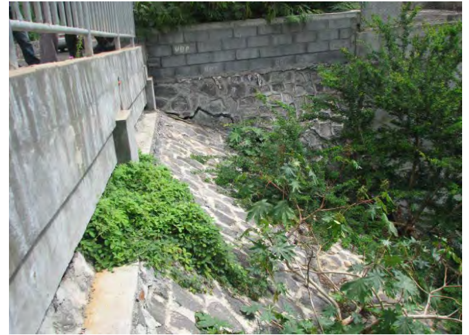
Cracks on stone wall
