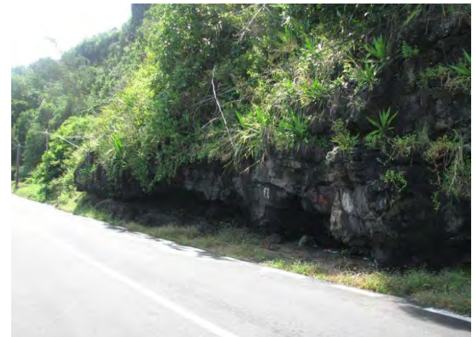
Clearance of the slope 2
