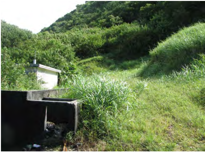
Full view of the collapse slope
