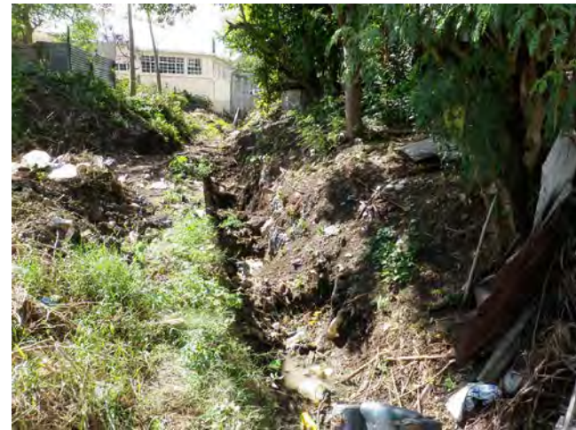
Toe of the landslide
