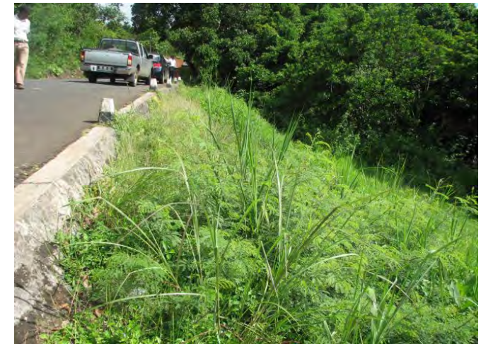
Road construction with fill
