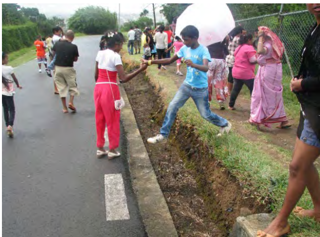
The back of the slope failure
