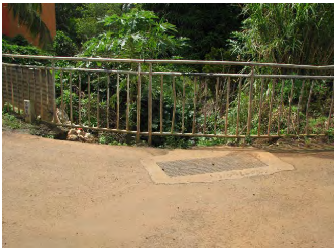
Full view of down stream
