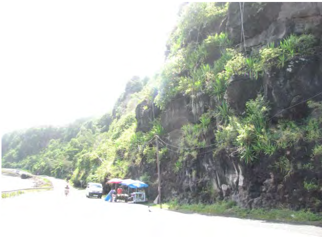
Full view of the slope 2
