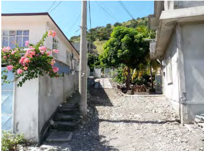
Full view of the slope from road
