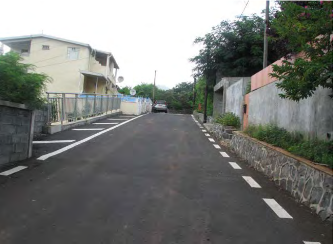
Full view (upper end of retaining wall)
