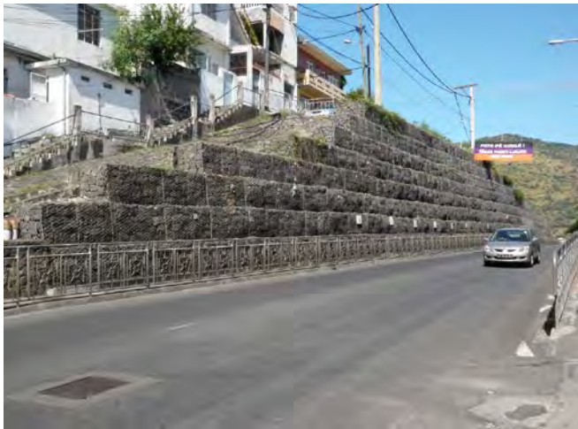
Full view of Gabion wall (East side)
