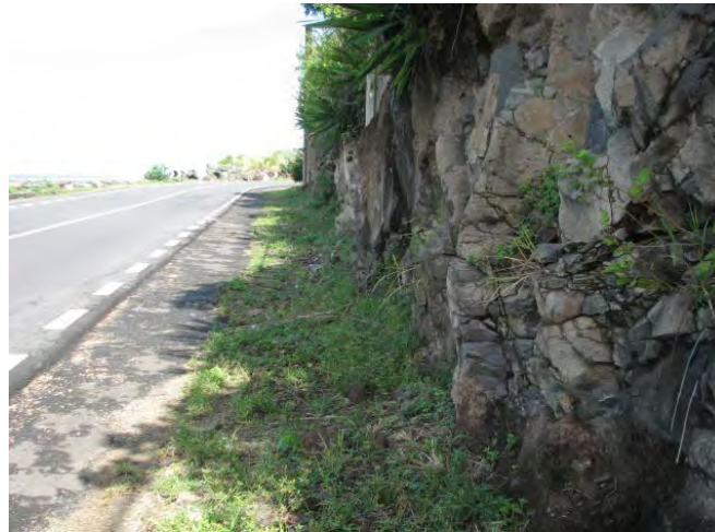
Clearance of the slope 1
