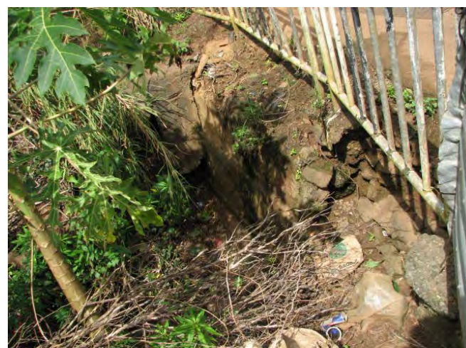
Outlet of downstream
