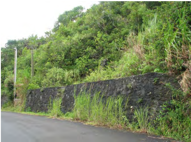
Full view (retaining wall)
