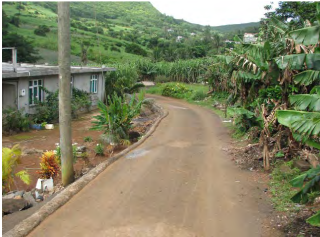
Full view of damage of retaining wall
