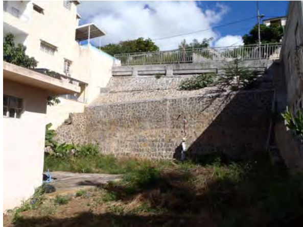
Ph-1 Full view (Retaining wall)
