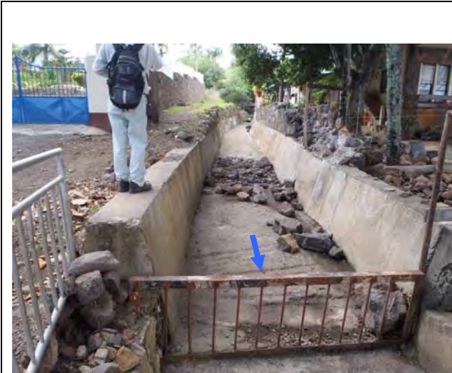
Ph-1 Full view of the channel works
