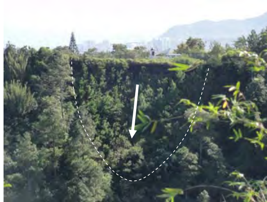
Ph-2 the slope failure B=35m, L=30m, D=2~3m
