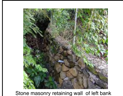
Stone masonry retaining wall of left bank
