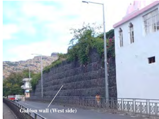
Ph-2 Full view of Gabion wall (West side)
