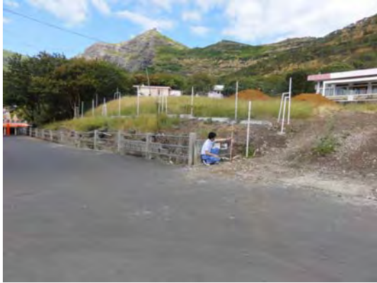
Ph-1 Full view of Embankments
