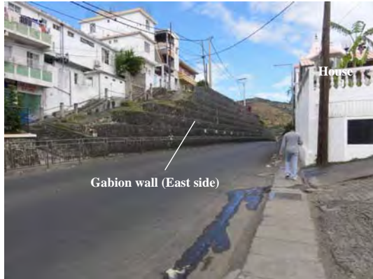
Ph-1 Full view of Gabion wall (East side)
