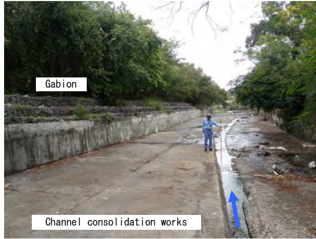
Ph-2 Stream of the channel consolidation works
