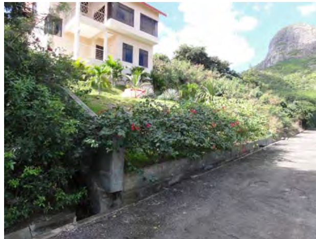
Ph-5 Toe of the slope
