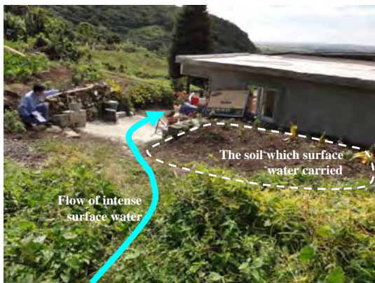
Ph-3 The course that the surface water flows through (1)
