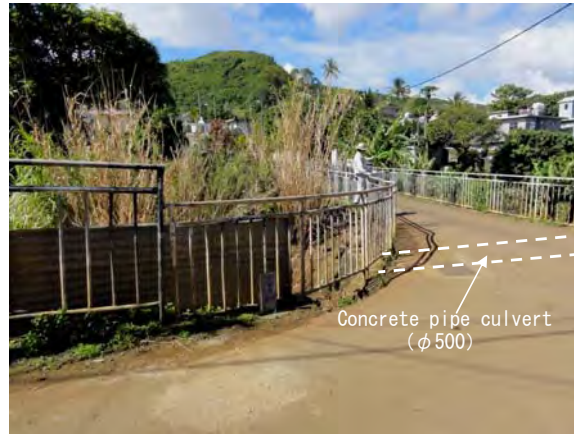
Ph-2 Full view (Down stream)
