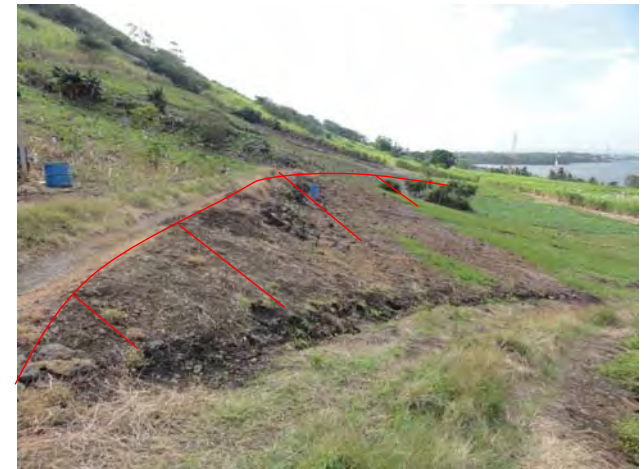
Ph-3 Scarps of the landslide upper part
