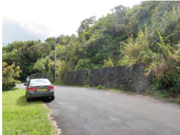
Ph-1 Full view (Retaining wall)
