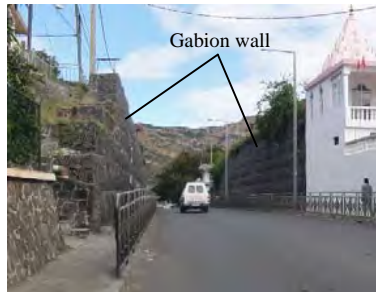
Ph-1 Full view of Gabion wall
