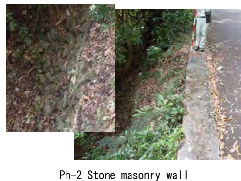
Ph-2 Stone masonry wall
