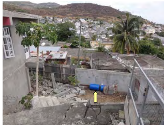
Ph-5 Direction of landslide movement
