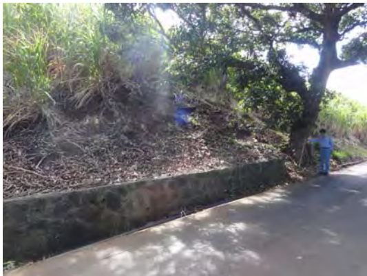
Ph-4 slope failure
