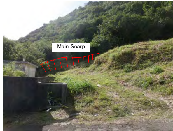
Ph-2 Collapse site
