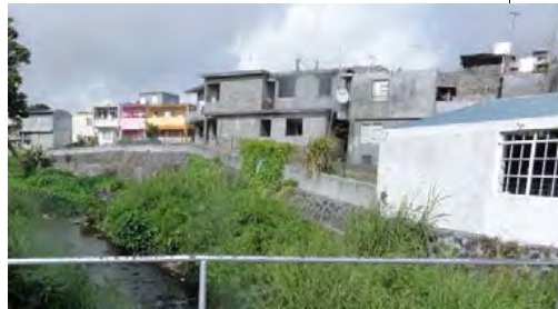
Stone masonry retaining wall (left bank)
