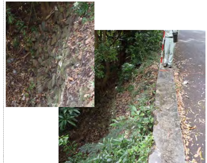
Ph-3 Stone masonry wall of the road shoulder (B-B' cross section)
