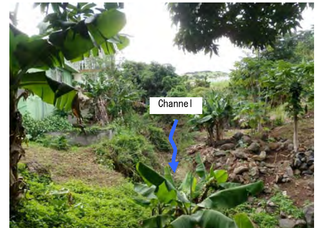
Ph-3 The upstream of channel works
