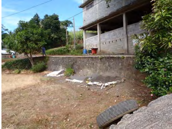
Ph-1 Full view (Retaining wall)
