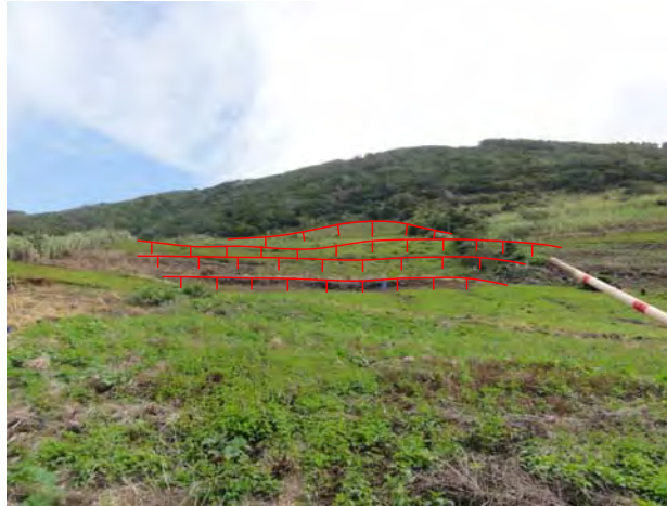
Ph-2 Scarps of the landslide upper part
