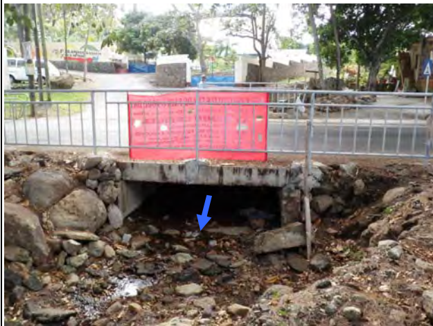
Ph-4 Box culvert
