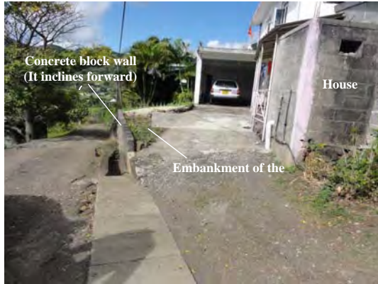
Ph-1 Full view of concrete block wall
