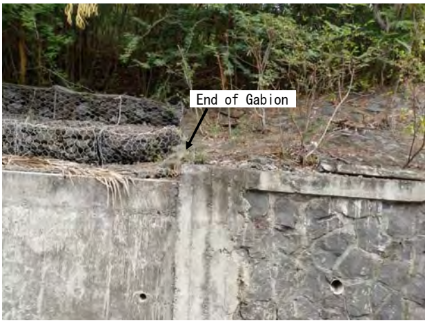
Ph-5 End of the gabion
