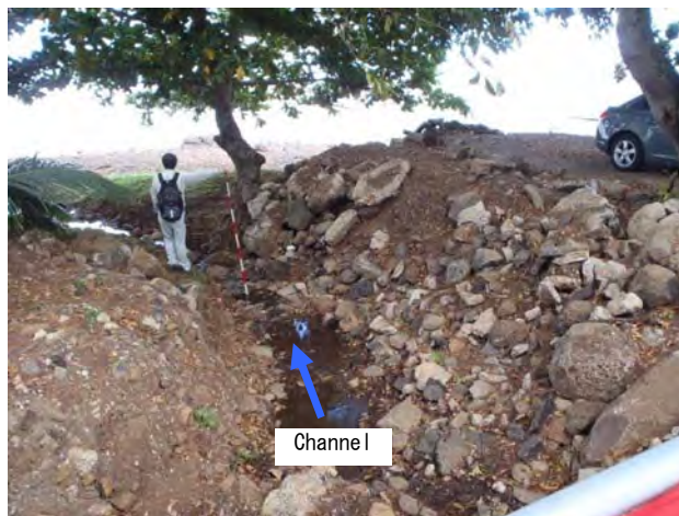
Ph-5 Discharged sediment at the mouth of stream
