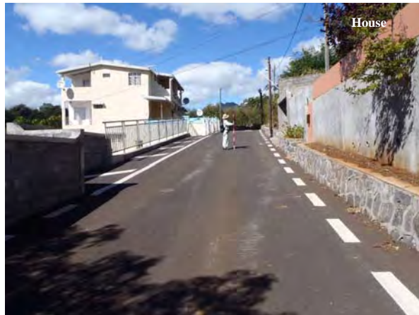
Ph-4 Full view (upper end of retaining wall)
