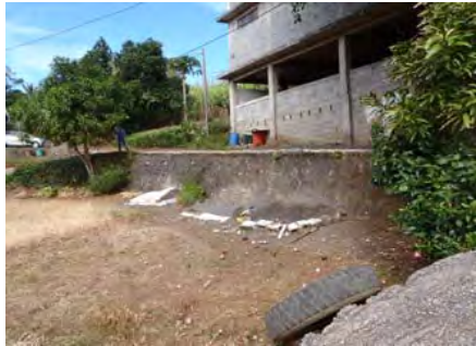
Ph-1 The retaining wall
