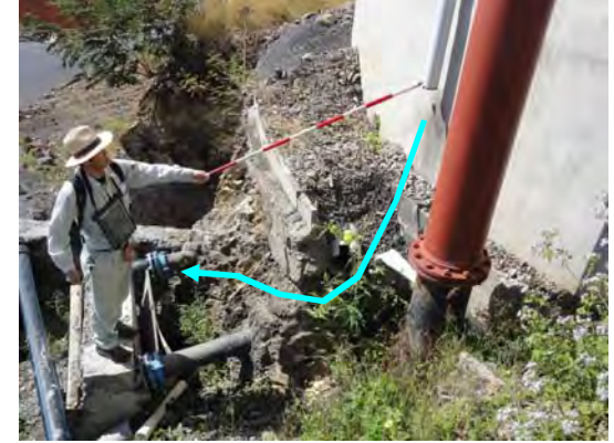
Ph-3 flow of surface water
