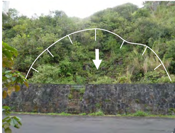
Ph-2 Trace of past slope failure
