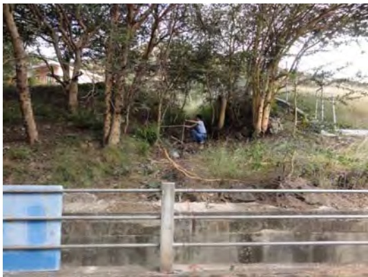
Ph-4 The Gully by flow of surface water
