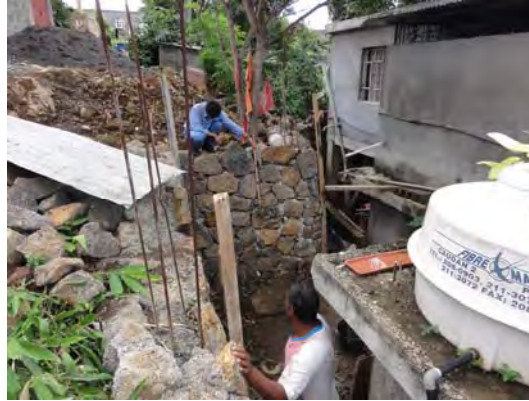
Ph-2 retaining wall
