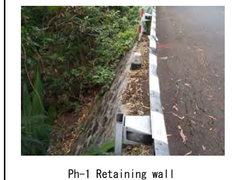
Ph-1 Retaining wall
