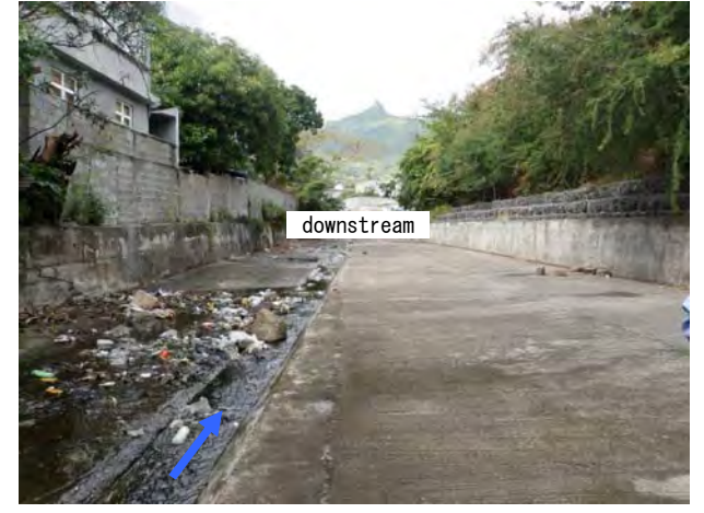
Ph-6 The channel works downstream
