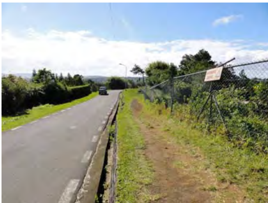
Ph-4 the back of the slope failure
