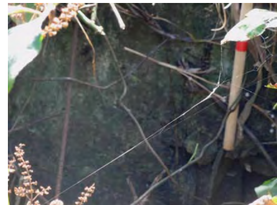
Ph-3 Concrete wall
