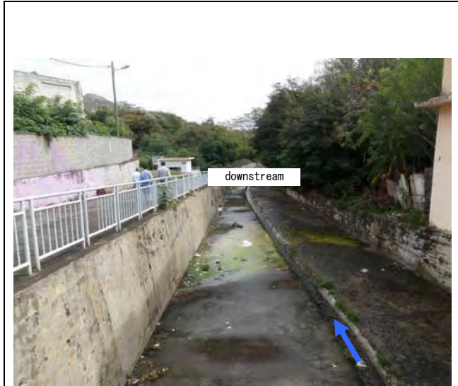
Ph-1 Full view of the channel consolidation works
