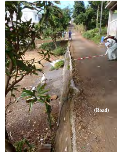
Ph-3 Retaining wall
