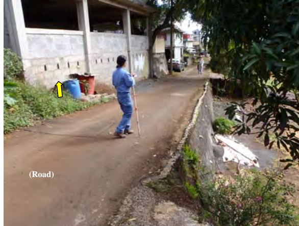
Ph-2 Retaining wall
