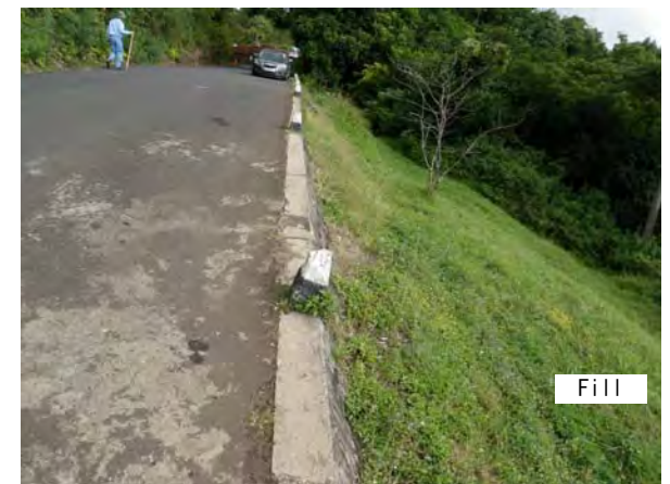
Ph-6 Road constructed with fill
