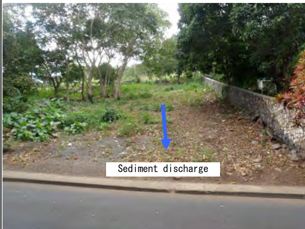
Ph-4 Slope where outflow of gravel and soil are expected
