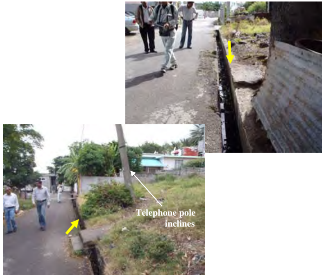
Ph-2 Retaining walls incline
