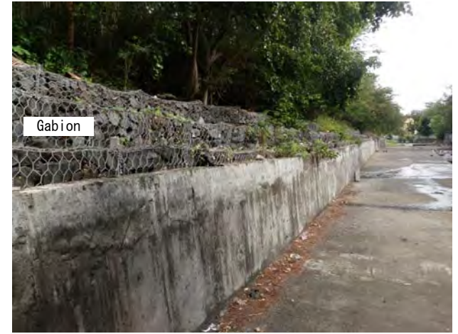
Ph-3 Gabion set up in channel consolidation works left bank
