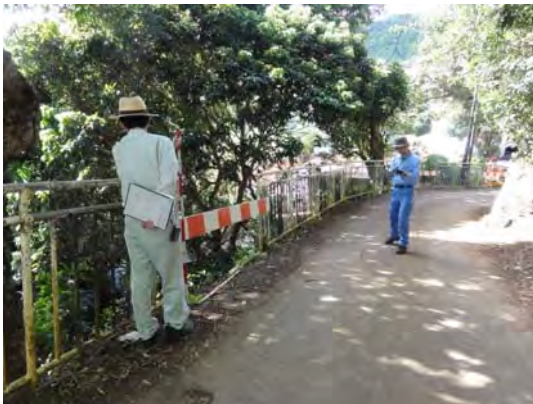
Ph-3 repaired road of another site
