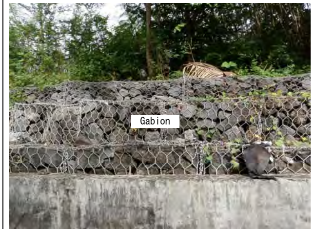
Ph-4 There is no damage
