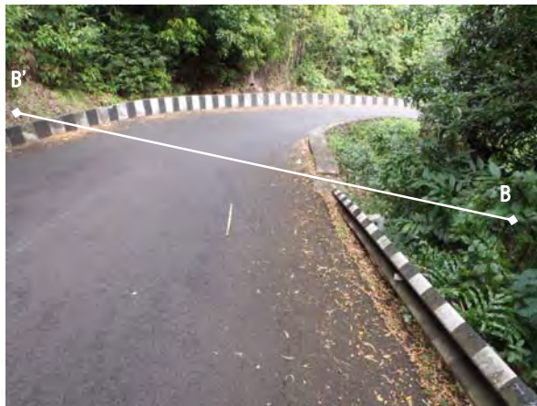
Ph-1 Full view (Cracks and subsidence on the road)
