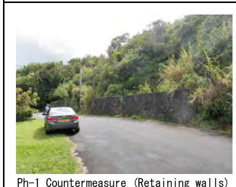
Ph-1 Countermeasure (Retaining walls)
