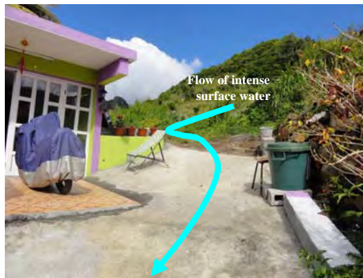
Ph-4 The course that the surface water flows through (2)
