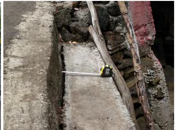
Photo 3.7.78 Opening between Road and Boundary Line
