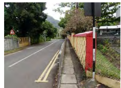
Photo 3.7.18 The Wall and Sidewalk facing Main Road (source:JET)
