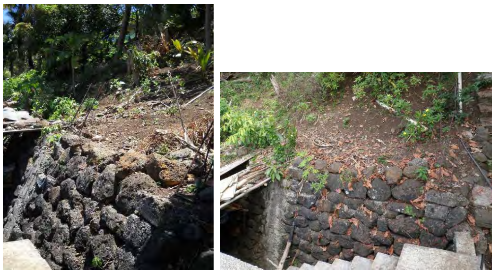
Photo 3.7.83 Masonry Retaining Wall behind House 19 (Left: 2011, Right: Present)
