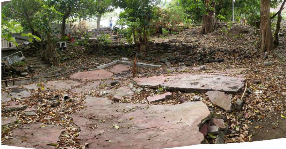
Photo 3.7.26 Deformation of the Concrete Foundation of Suspected House Remains
