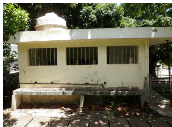
Photo 3.7.13 Lavatory beside School (House No.9) (source:JET)
