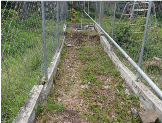
Photo 3.7.9 Vertical Displacement beside Extensometer(5)
