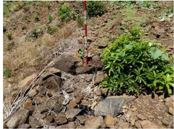
Photo 3.7.67 Deformations around Elevation 45m (Current Condition)
