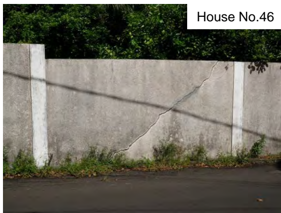
Photo 3.7.55 Cracks in the Wall
