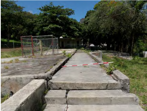
Photo 3.7.5 Steps to the School Building Foundation (East Side)
