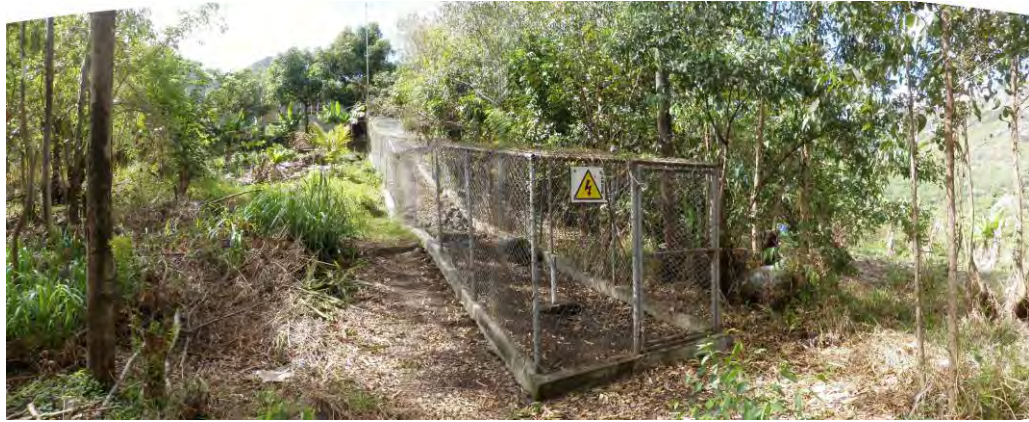
Photo 3.7.34 Extensometer E(1) (Shot from below) (source:JET)
