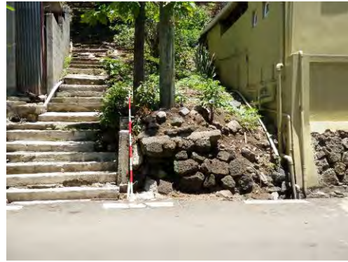
Photo 3.7.87 Masonry Retaining Wall in front of the Road (source:JET)
