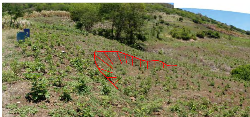
Photo 3.7.73 Collapse at the Head of a Stream (source:JET)
