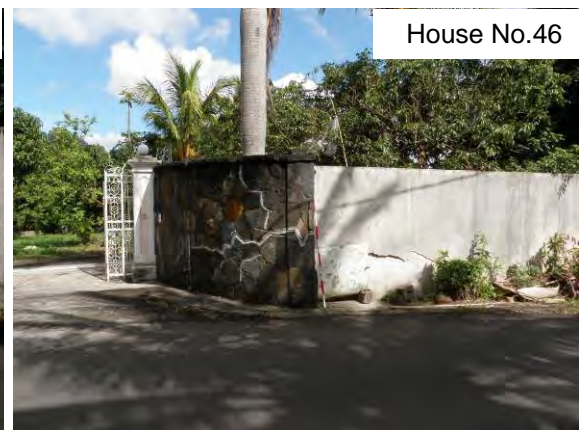
Photo 3.7.56 Cracks in the Wall (Entrance)
