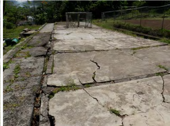
Photo 3.7.6 Floor of the School Building Foundation (West Side)
