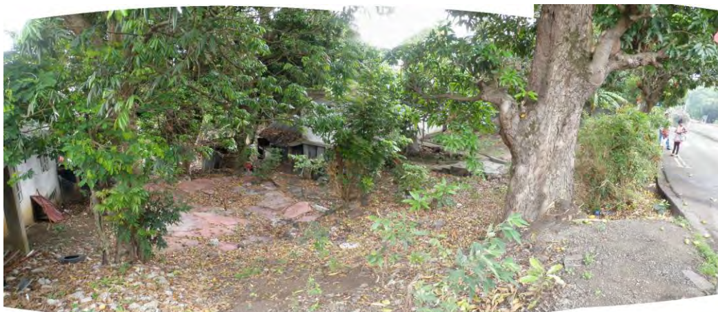
Photo 3.7.25 Deformation of the House in front of the School (source:JET)
