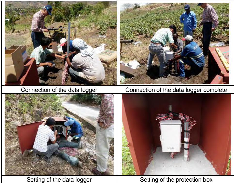
Photo 3.6.2 Installation of the Pipe Strain Gauge (source: JET)
