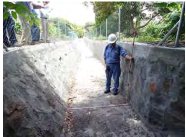
Completed Countermeasure Work 【River Type-3】, 12 th Dec. 2014
