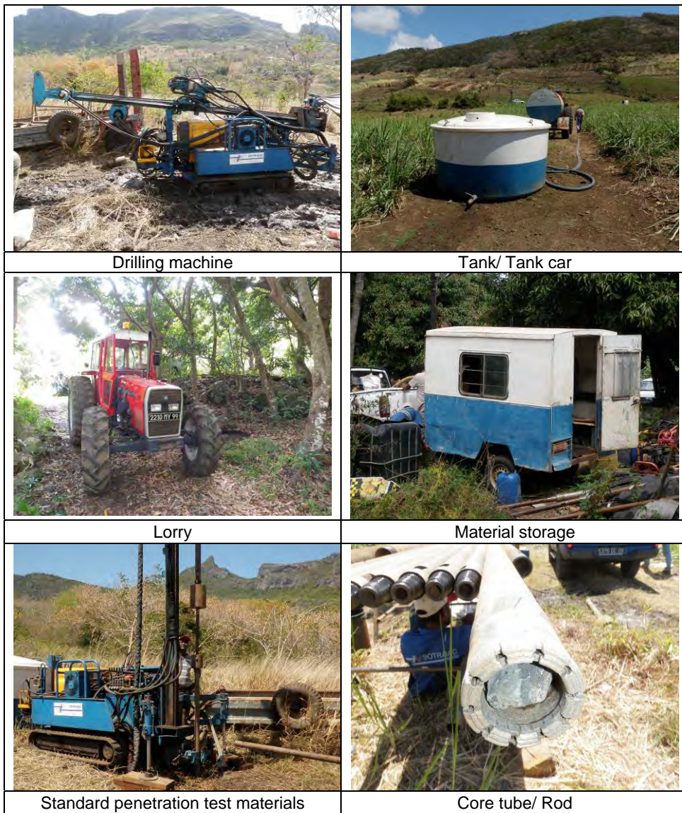
Photo 3.6.1 The Drilling Machines and Materials (source: JET)
