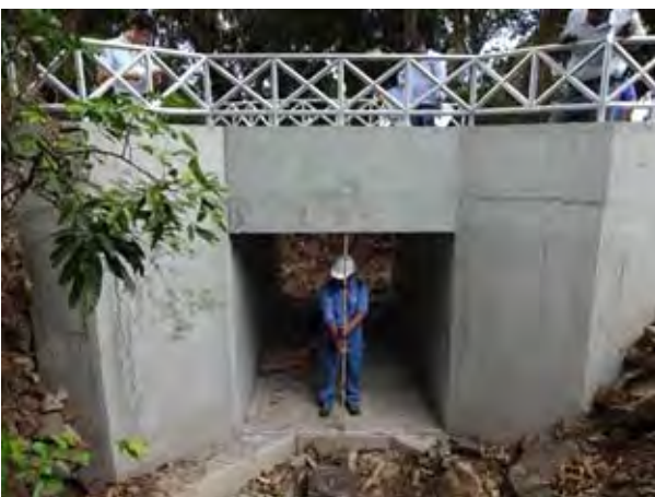
Completed Countermeasure Work 【Bridge Type-3】, 12 th Dec. 2014
