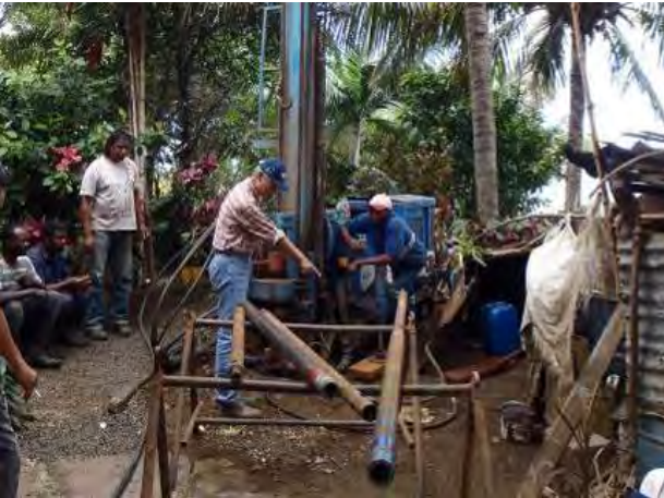
Boring Survey (Quatre Soeurs), 2 nd Oct. 2012
