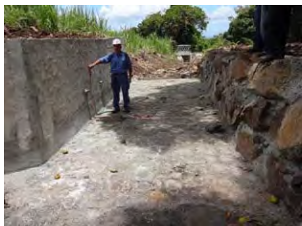
Completed Countermeasure Work 【Horizontal Drainage】, 12 th Dec. 2014
