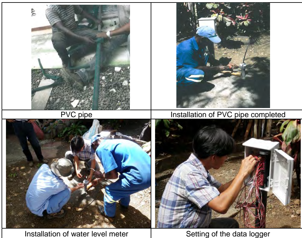
Photo 3.6.4 Installation of Water Level Meter (source: JET)
