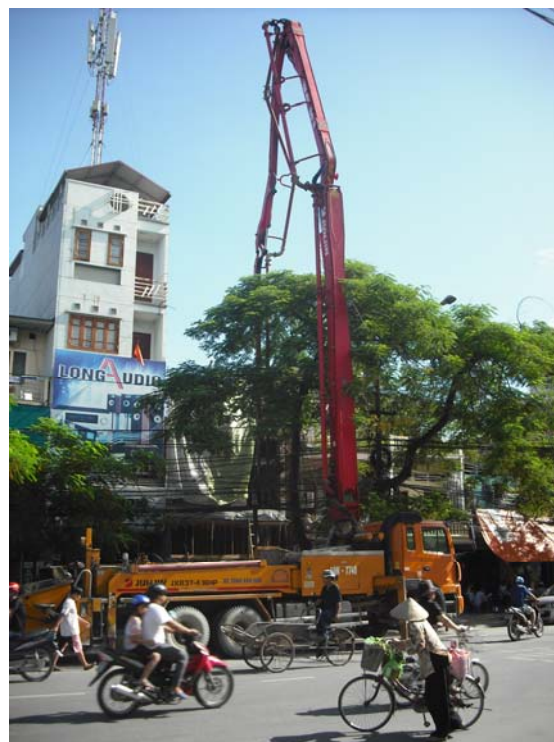
Photo 2-2-4 Working Concrete Pumping Truck (Hai Phong City)
