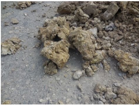
Cement Stabilized Base course of Sand + Gravel Cement Stabilized Sub-base of Clay
