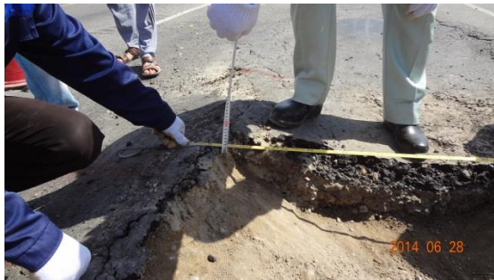
⑤ Pavement Thickness 2cm
