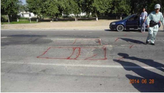
① Excavation Survey
