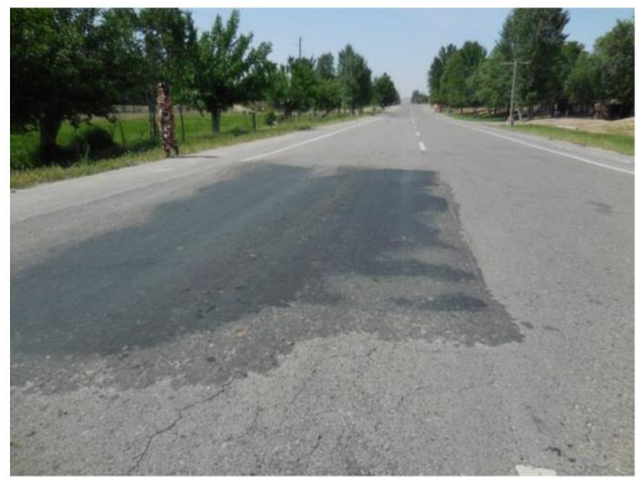
Repair by Cold Mixture at AC Pavement Defect Location
