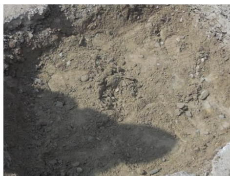
Cement Stabilized Base course of Sand + Gravel
