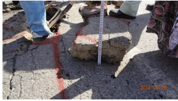
② Pavement Thickness 12cm (5cm+7cm)
