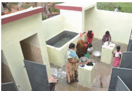
Washing facilities are provided
