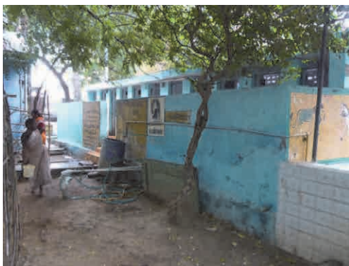
View of the community toilet
