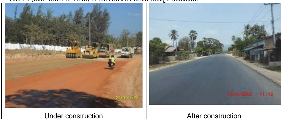
Figure 3.6 Road Widening in Myawaddy-Thingannyinaung Section
