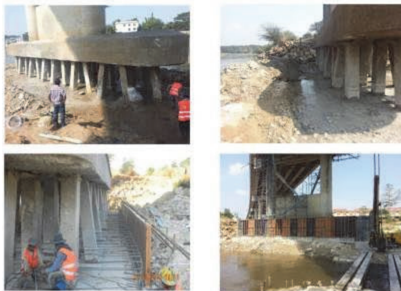
Figure 3.11 Pier (P7) Repair Work for the First Thailand – Myanmar Friendship Bridge
