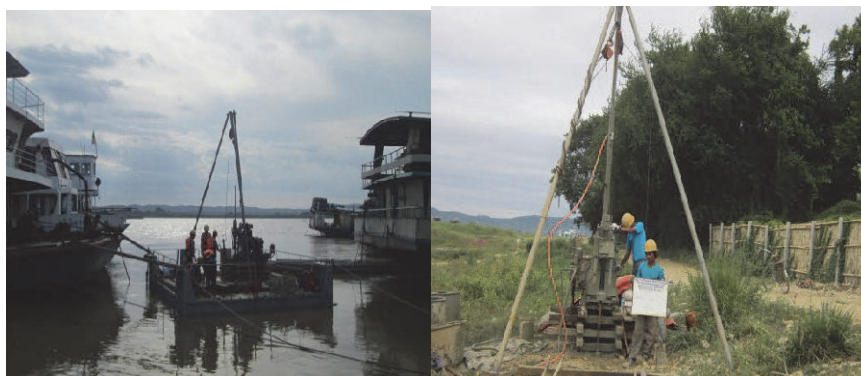
Figure 5.9 Condition of Soil Investigation on Water and on Land
