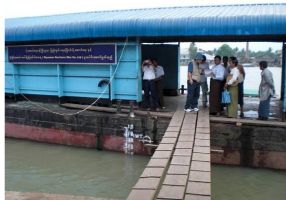
Photo C.1.50 Bogalay Station Station Pontoon and Bridge
