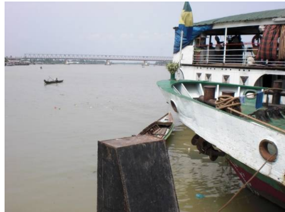
Photo C.1.40 View Bridge from Station
