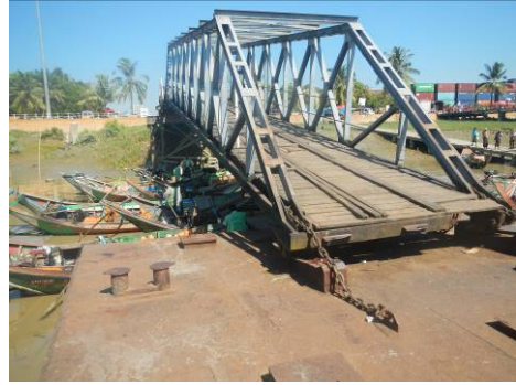
Photo 8 - Steel bridge and sponson
