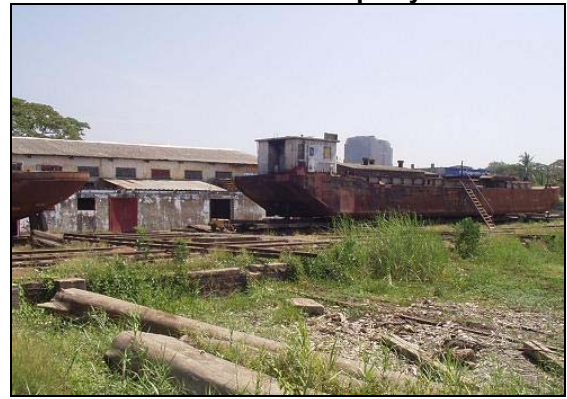
Photo C.2.18 No.6 Side Slipway
