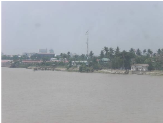
Photo B.4.51 Monkey Point Signal Station
