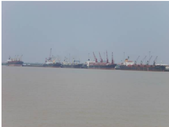
Photo B.4.49 Thilawa Port 5 vessels alongside to Thilawa Port Pier
