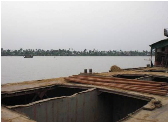
Photo C.1.53 Moored Barge at the Station Pontoon
