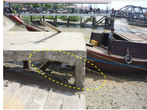
Photo 4 - concrete damage
