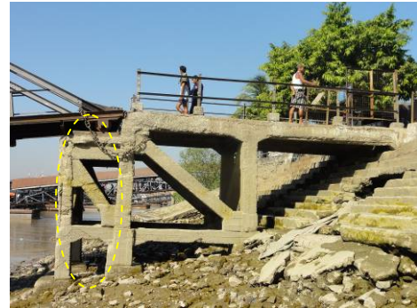
Photo 4 - Abutment damage
