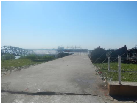
Photo 2 - Abutment Corner damage
