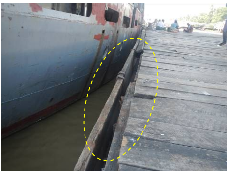
Photo 3 - Decking Damage
