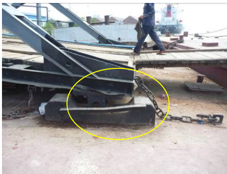
Photo 3 - Roller wheel is missing
