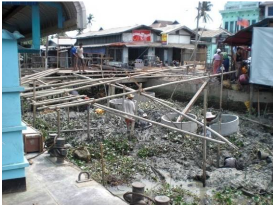
Photo C.1.39 Terminal building and Bridge are under construction
