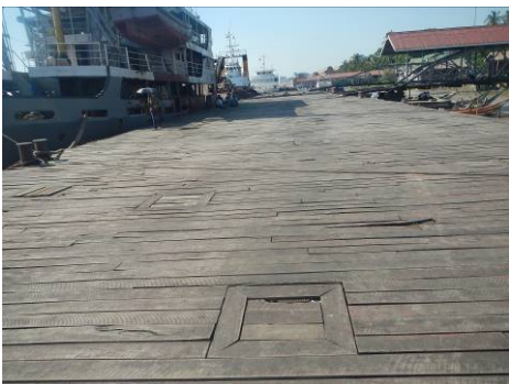
Photo 3 - Pontoon timber floor
