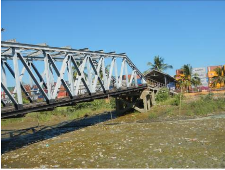
Photo 7 - Steel bridge and Pier
