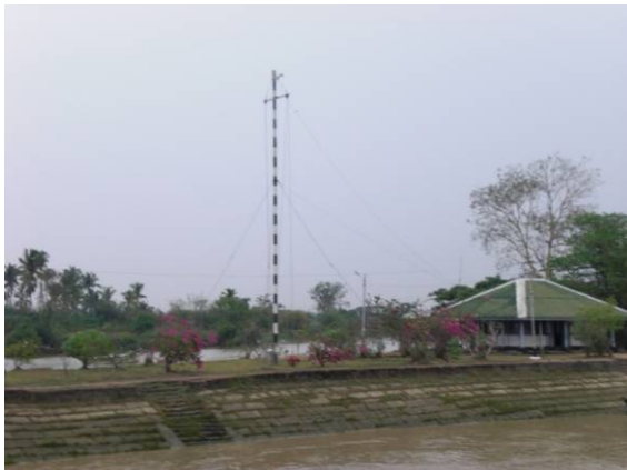
Photo C.1.11 Signal Station of Canal
