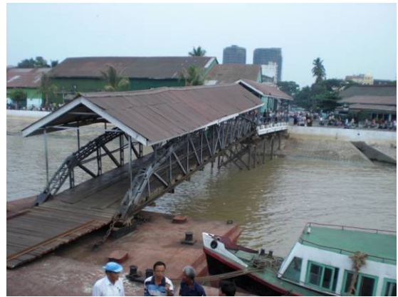
Photo C.1.2 Lan Thit Jetty ,Yangon Bridge and Sponcer
