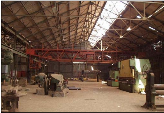
Photo C.2.11 Plating and angle shop
