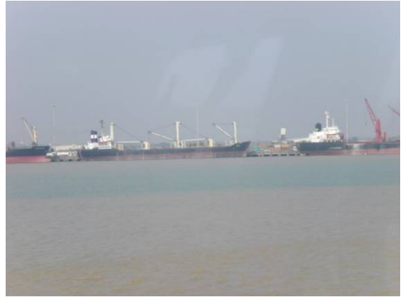
Photo B.4.20 5 vessels berthing at Thilawa Port
