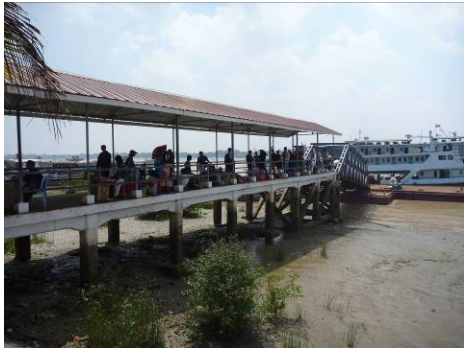
Photo 1 - Porter way C.G.I roofing is added
