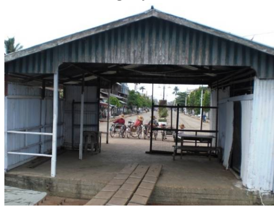
Photo C.1.48 Bogalay Station Terminal house and bridge
