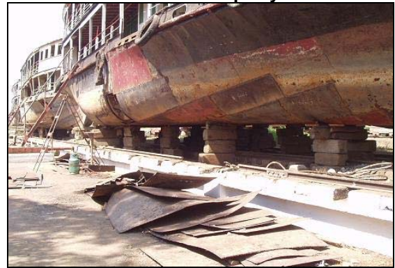
Photo C.2.20 Renewed Bottom Shell Plates
