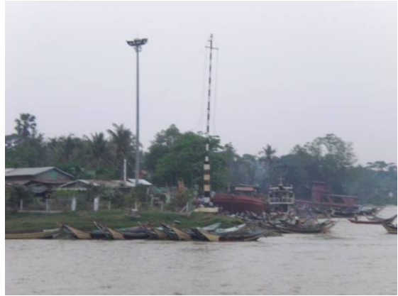
Photo C.1.8 Signal Station of Canal In case dangerous situation by low tide, Black Ball in daytime, Red Light in night is hoisted the poll.
