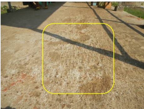
Photo 3 - Surface delaminated
