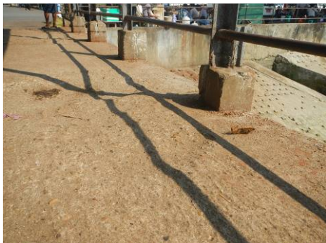
Photo 3 - Surface delaminated
