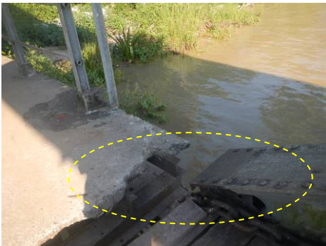
Photo 2 - Corner damage
