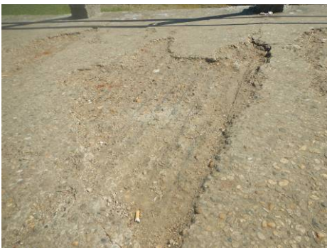
Photo 3 - Slab concrete surface
