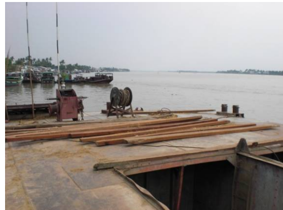
Photo C.1.54 Moored Barge at the Station Pontoon
