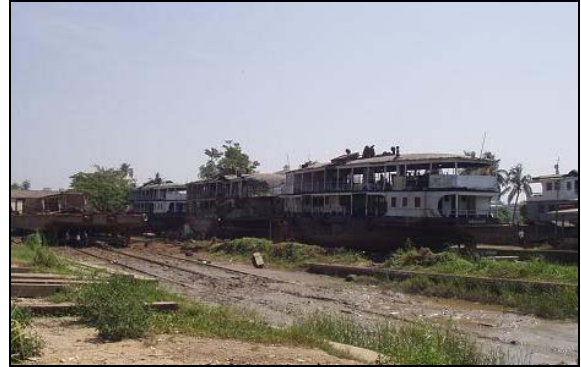
Photo C.2.16 No. 5 & No. 7 Slipway
