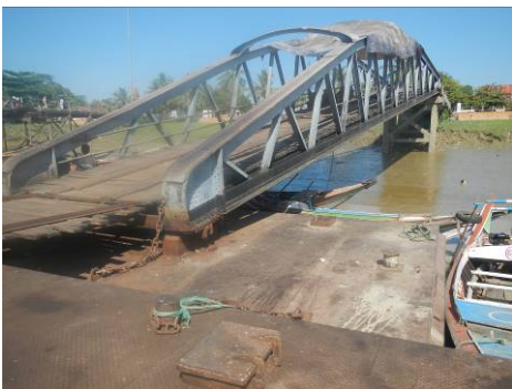
Photo 3 - Steel Bridge and Sponson
