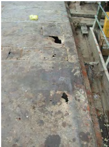
Photo 2 (Hole of upper plate at Pontoon)
