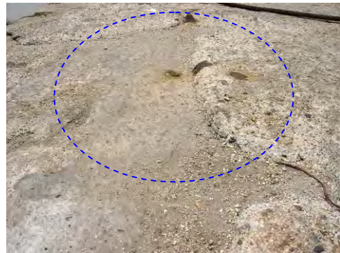
Photo 4 - Surface of concrete
