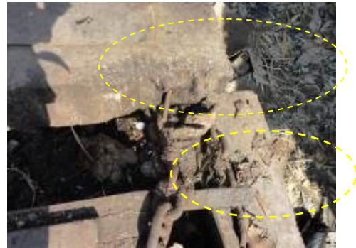
Photo 6 - Connection of steel bridge & abutment
