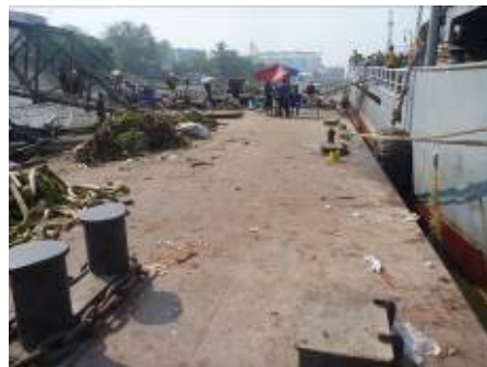
Photo 6 - Debris on the pontoon ( reason of damage)
