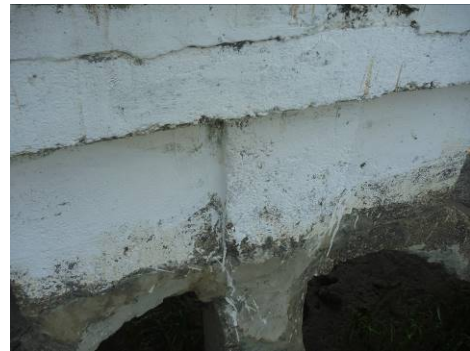
Photo 4 - Repaired beam and column
