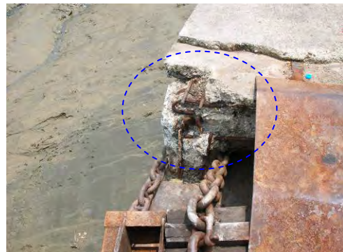
Photo 6 - Edge of Pier
