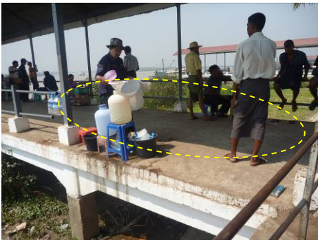
Photo 2 - Handrail missing
