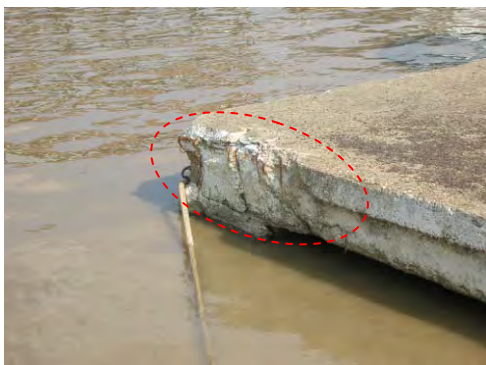
Photo 3 - Edge of beam
