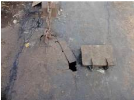
Photo 3 - Pontoon Top cover damage
