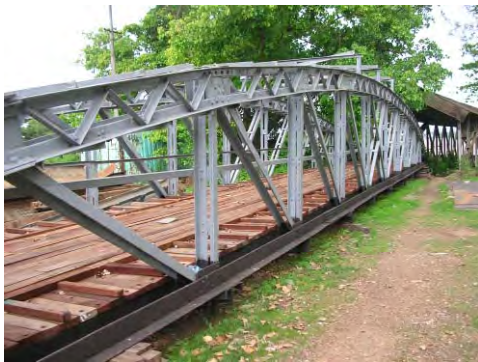
Photo 2 - New Bridge under construction
