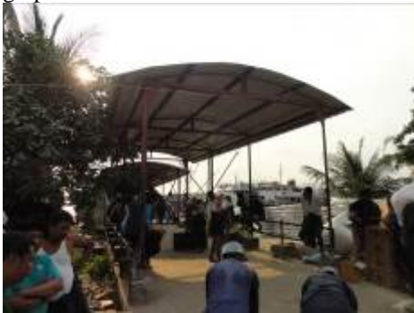
Photo 1 - New pier Added roof
