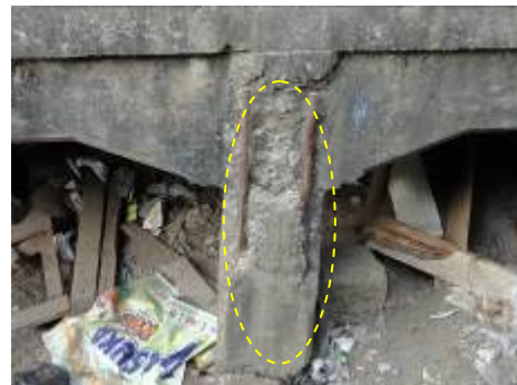
Photo 5 - Column damage
