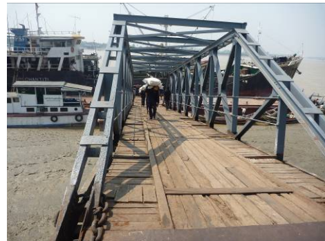
Photo 5 - New painted steel bridge with timber decking
