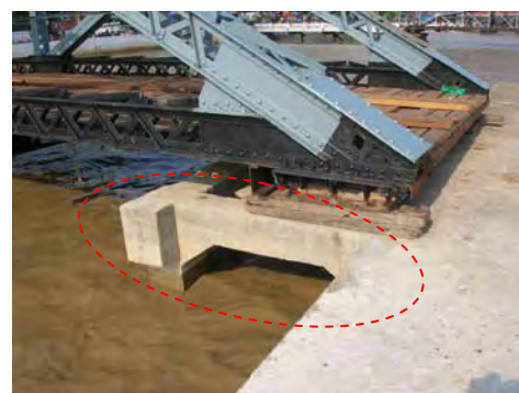
Photo 6 - Reference: New Concrete
