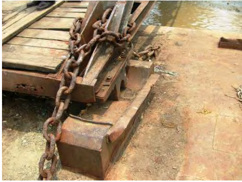
Photo 7 - Support of Bridge
