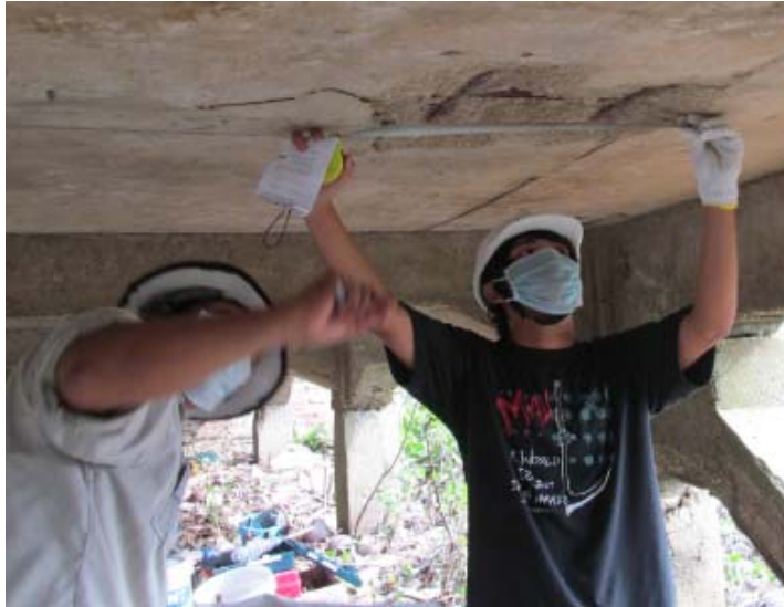
Photo 13.4.3 Spalling and Delamination of Concrete Cover
