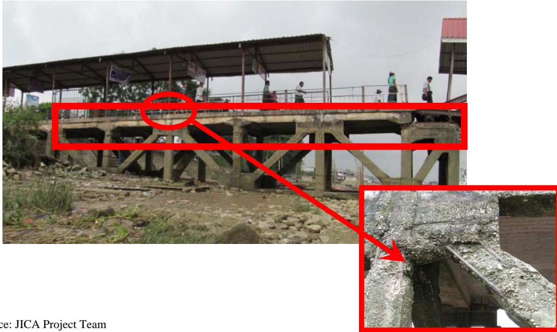
Photo 13.4.12 Area in Poor Condition (Dalla Jetty)
