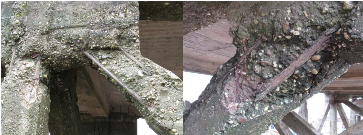
Photo 13.4.4 Spalling and Delamination of Concrete Cover
