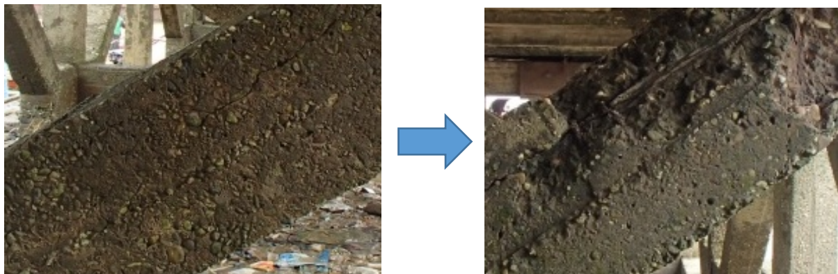
Photo 13.4.11 Chipping Concrete Cover and Exposing Rebar
