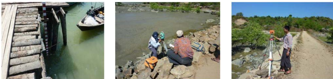
Figure 11.8.13 Setting Staff Gauges and Survey of Control Points
